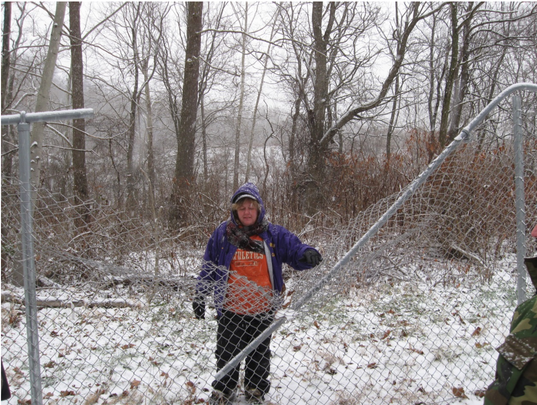
BUR 12/2013. PL-6. Damaged fence east of perimeter sign P11.
