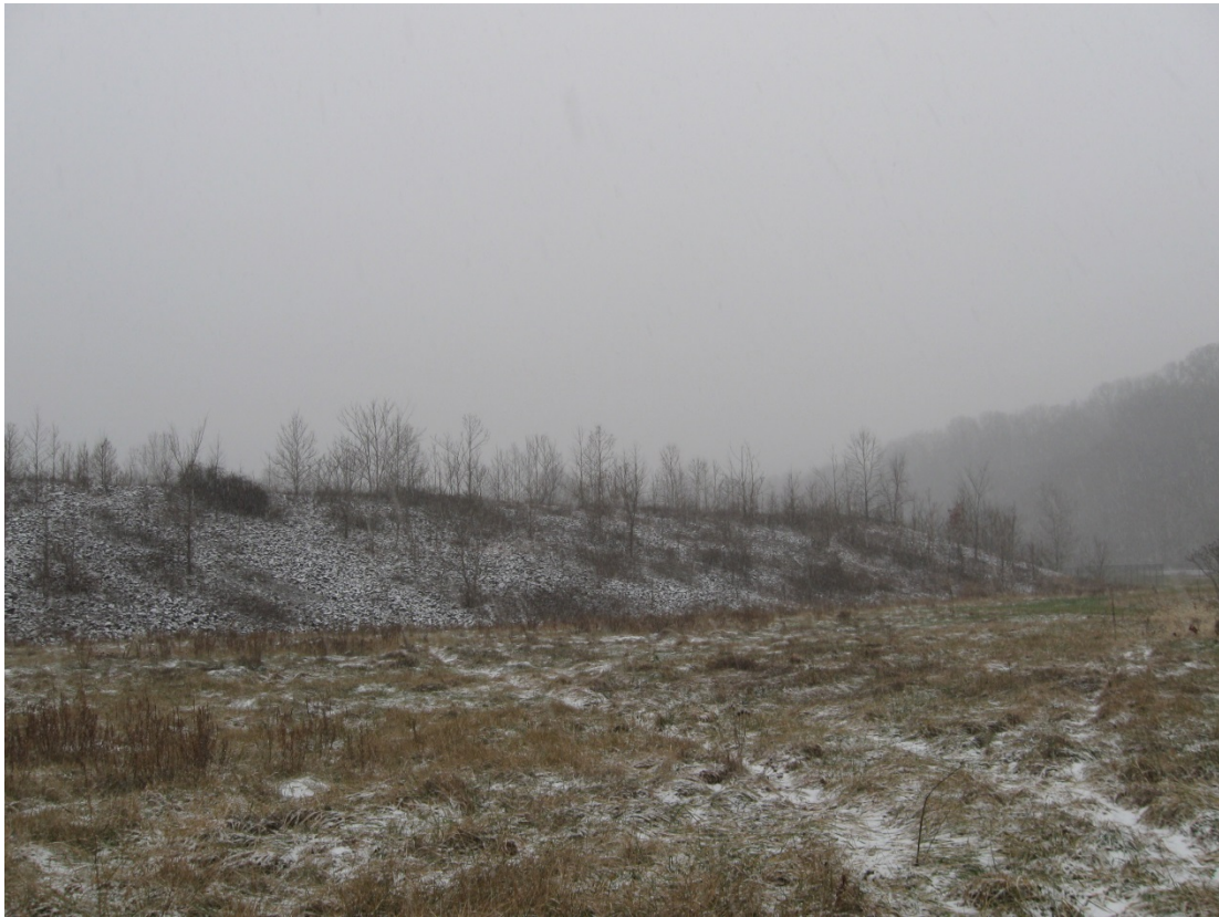
BUR 12/2013. PL-10. Northeast face of disposal cell.
