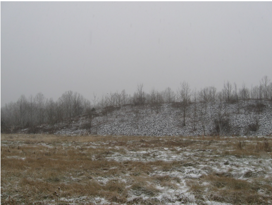
BUR 12/2013. PL-9. Northeast face of disposal cell.
