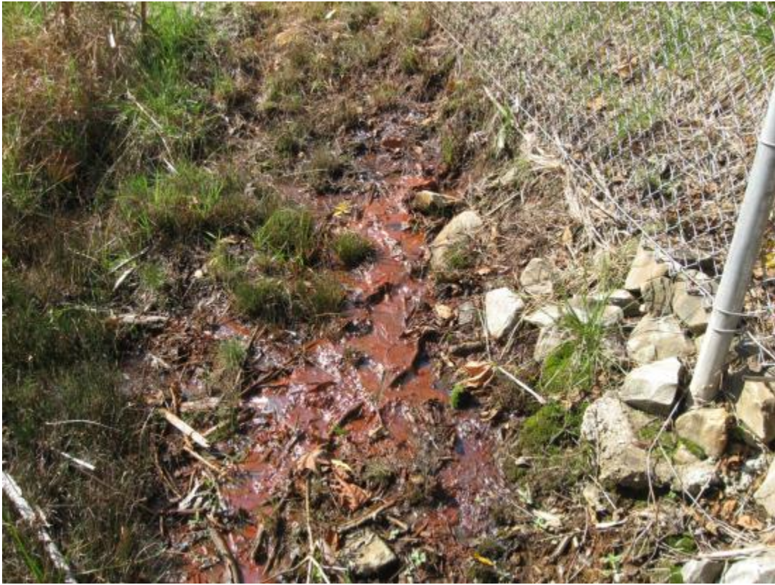
BUR 10/2012. PL-9. Active seep; north fence.
