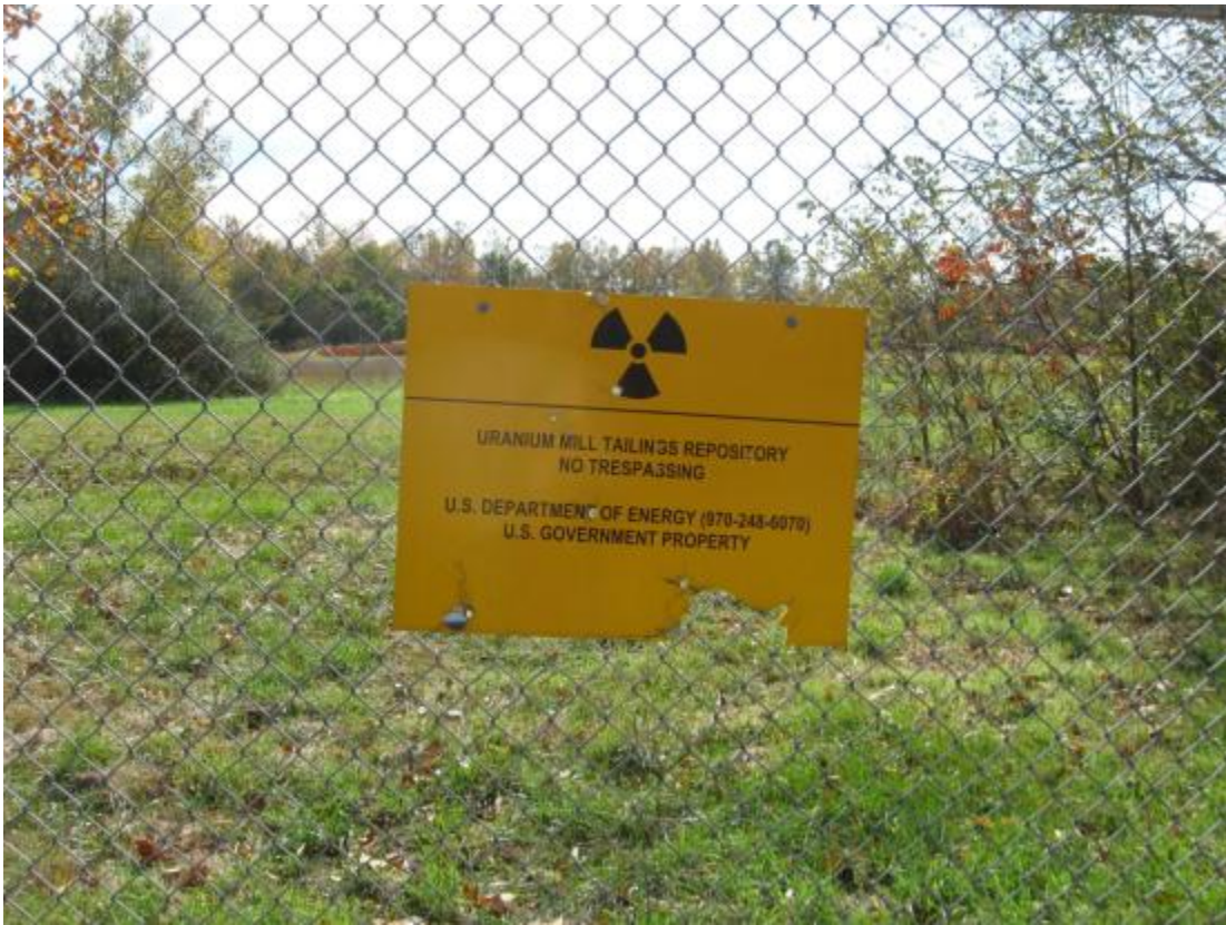
BUR 10/2012. PL-3. Bullet holes in perimeter fence sign P4.
