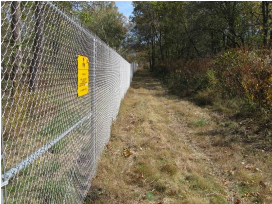
BUR 10/2012. PL-2. Southwest fence line.
