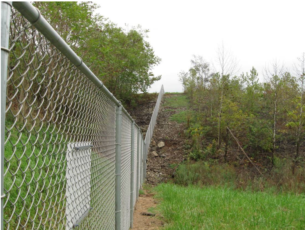
BUR 10/2011. PL-2. Vegetation cleared from perimeter fence.
