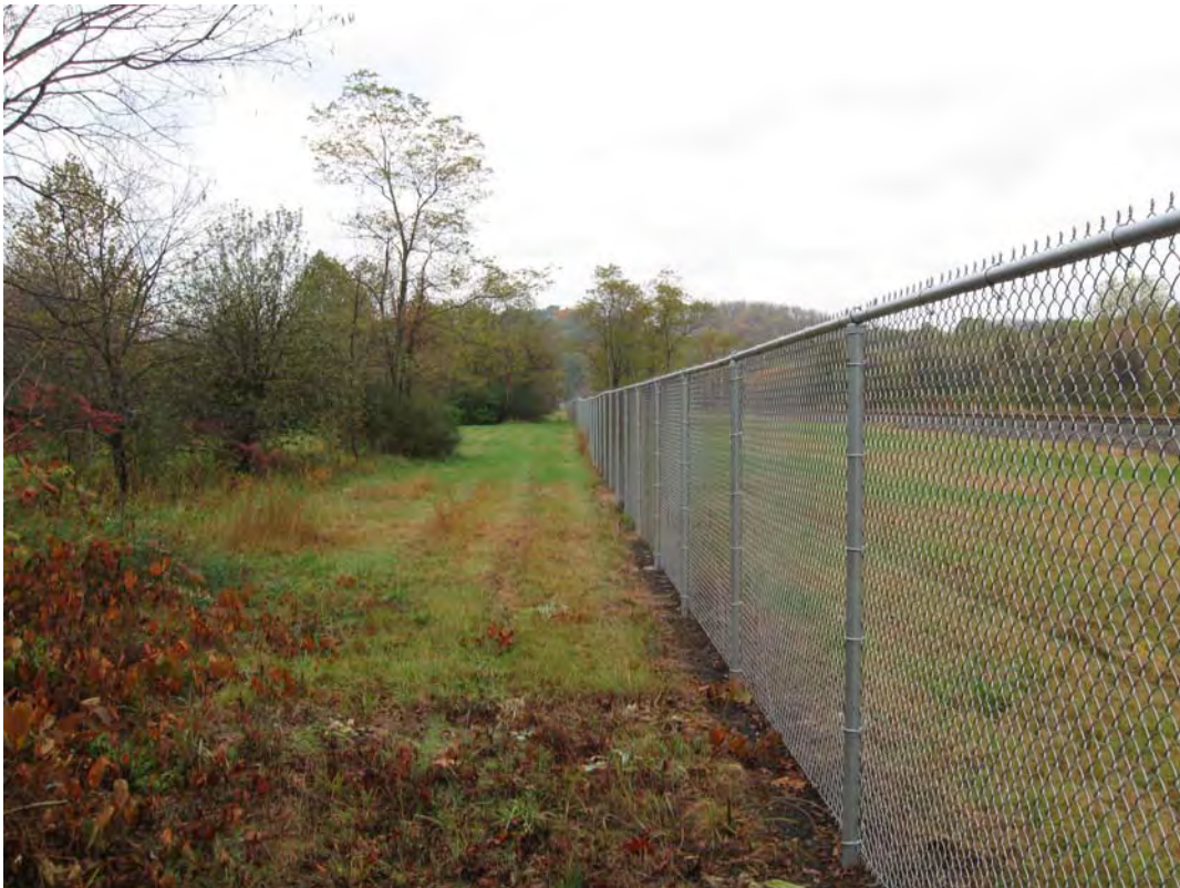
BUR 10/2010. PL-2. View down the inside of the north perimeter fence.
