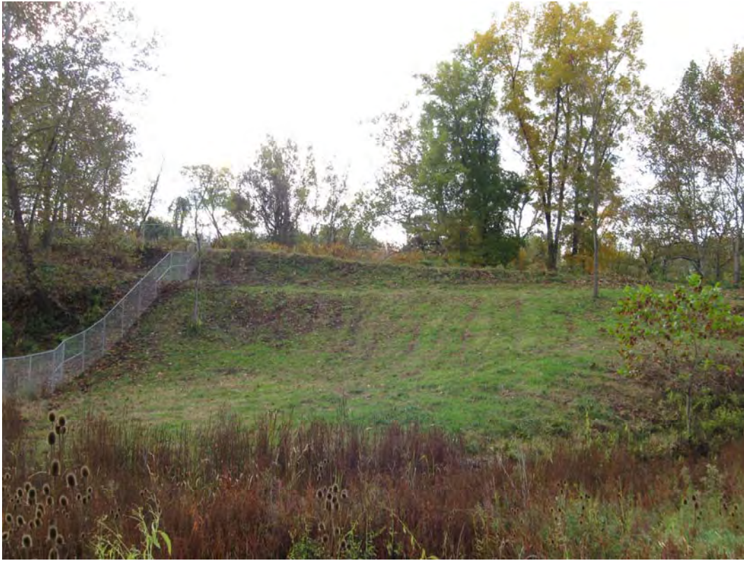
BUR 10/2010. PL-5. Looking south toward seeded slope.
