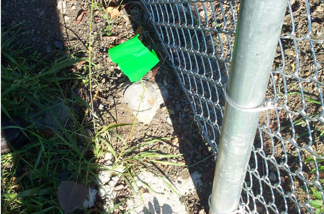
BUR 9/2007. PL-3. Boundary monument BM-5, damaged.
