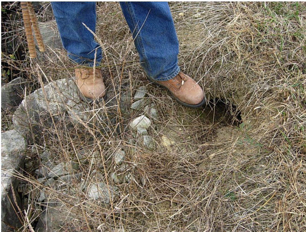
CAN 10/2008. PL-3. Animal burrow along edge of the disposal cell and diversion channel.
