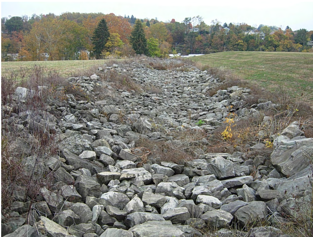
CAN 10/2008. PL-4. Riprap-armored diversion ditch northwest of the disposal cell.
