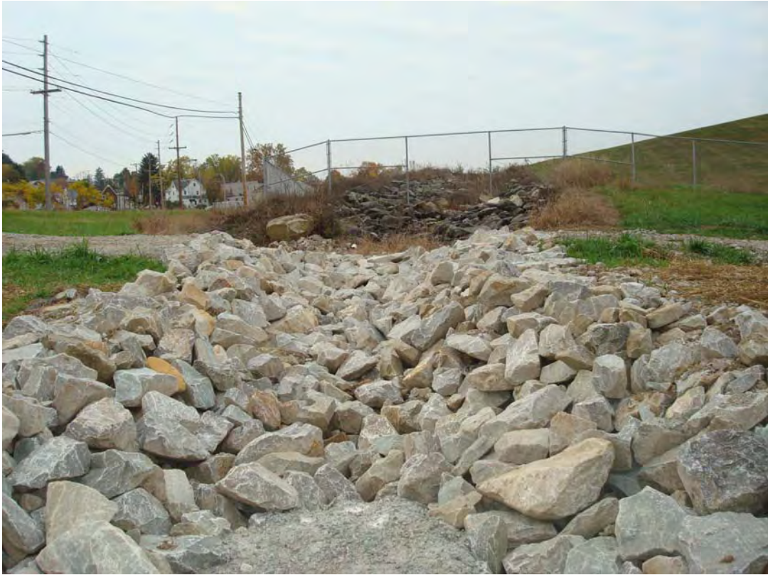
CAN 10/2008. PL-5. Riprap restoration at outlet to the east diversion channel.
