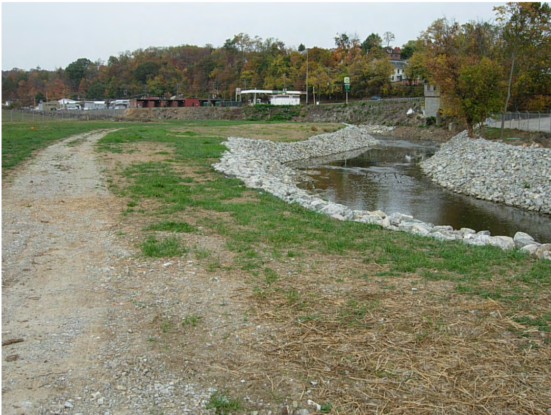
CAN 10/2008. PL-6. Completed stream bank stabilization work west of Strabane Avenue Bridge.
