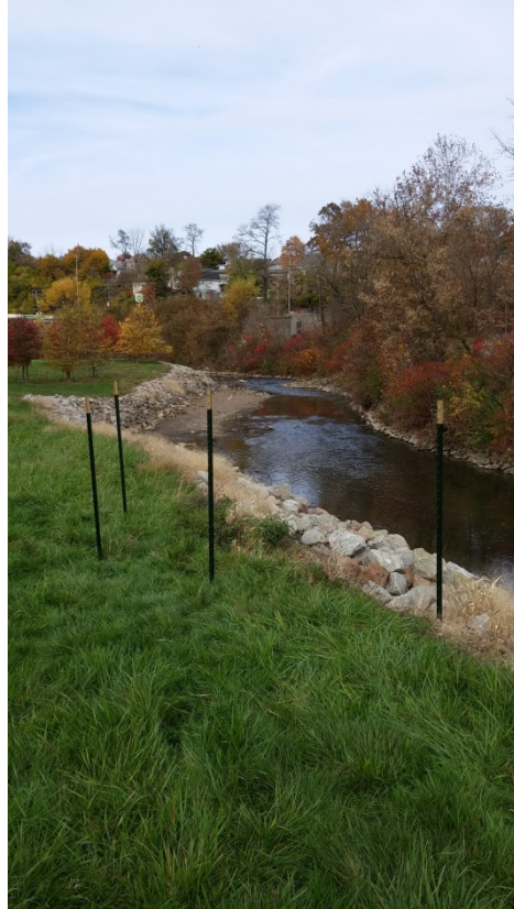
CAN 10/2015. PL-13. T-posts installed around erosion area.
