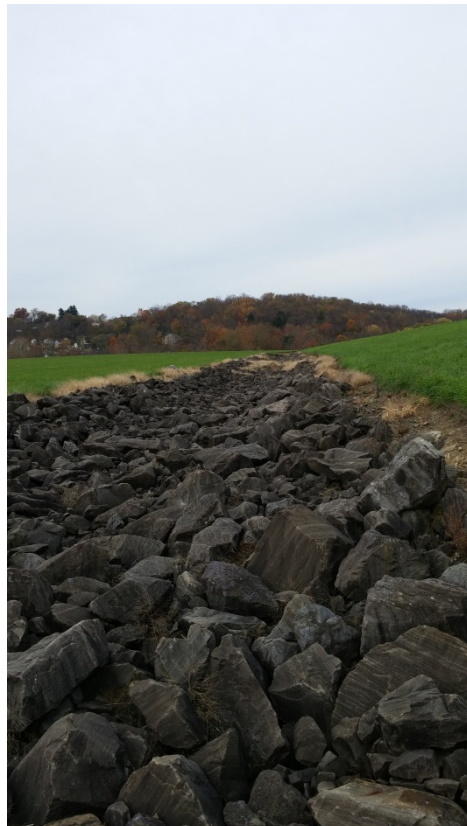
CAN 10/2015. PL-10. Armored diversion ditch on the southeast side of the disposal cell.
