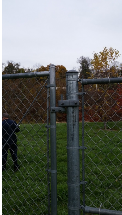
CAN 10/2015. PL-5. Repaired hinge on northeast vehicle gate.
