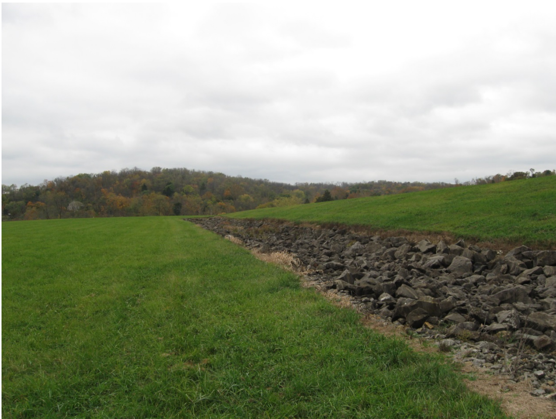
CAN 10/2014. PL-8. Riprap-armored diversion ditch.
