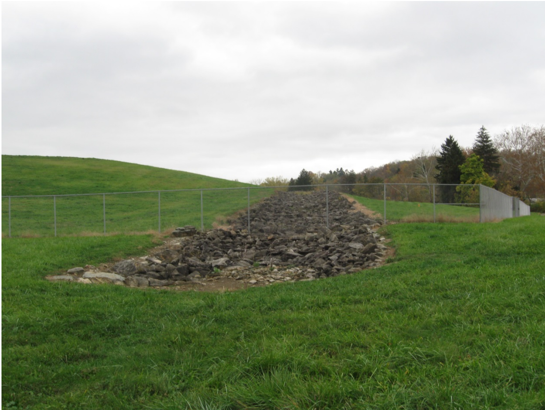
CAN 10/2014. PL-7. Riprap-armored diversion ditch.
