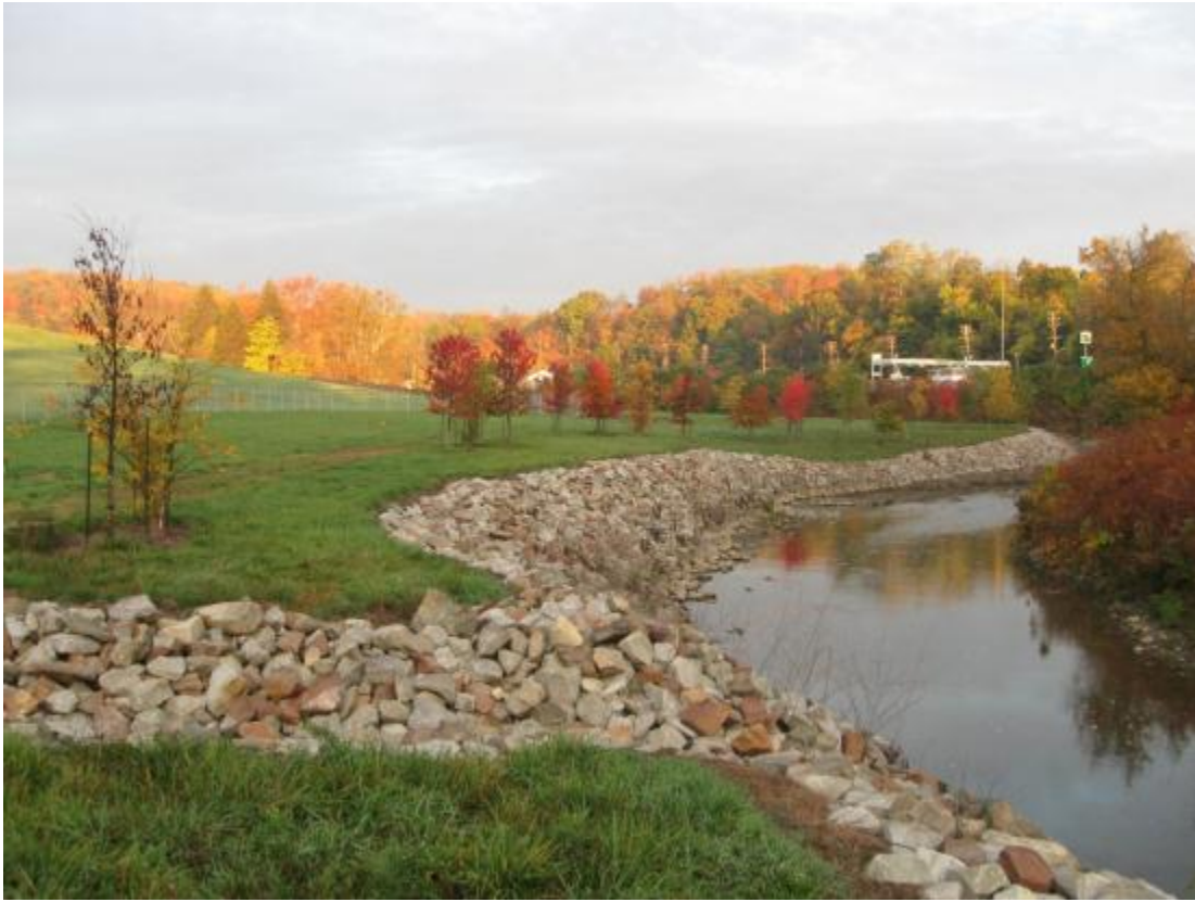
CAN 10/2012. PL-1. Riprap-armored stream bank.
