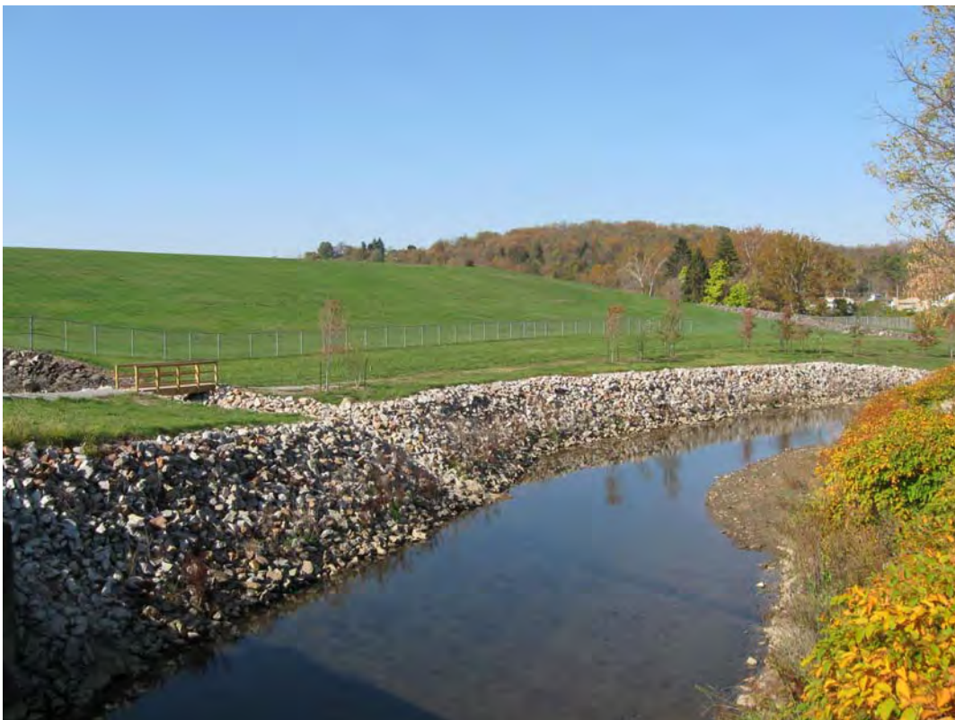
CAN 10/2010. PL-8. Riprap armored stream bank along floodplain area.
