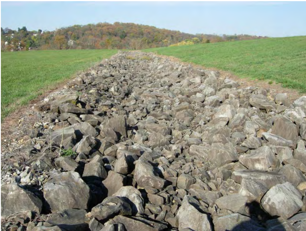
CAN 10/2010. PL-5. Riprap armored diversion ditch.
