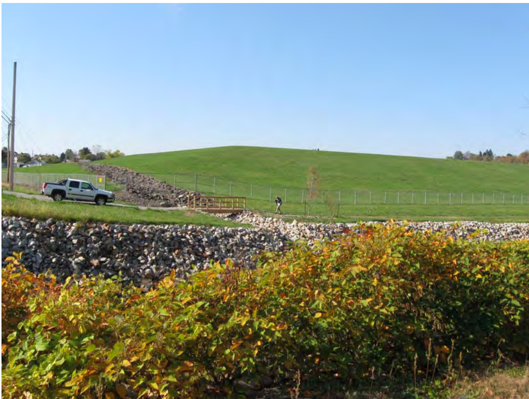
CAN 10/2010. PL-2. Footbridge across a riprap armored diversion ditch.
