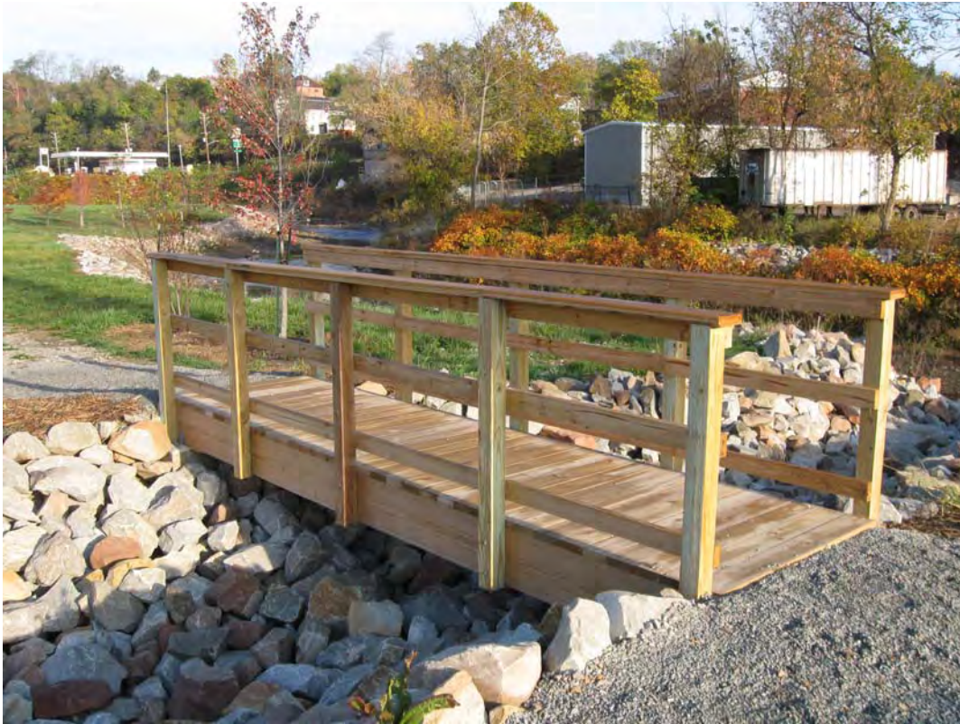
CAN 10/2010. PL-1. Newly installed footbridge across a riprap armored diversion ditch.
