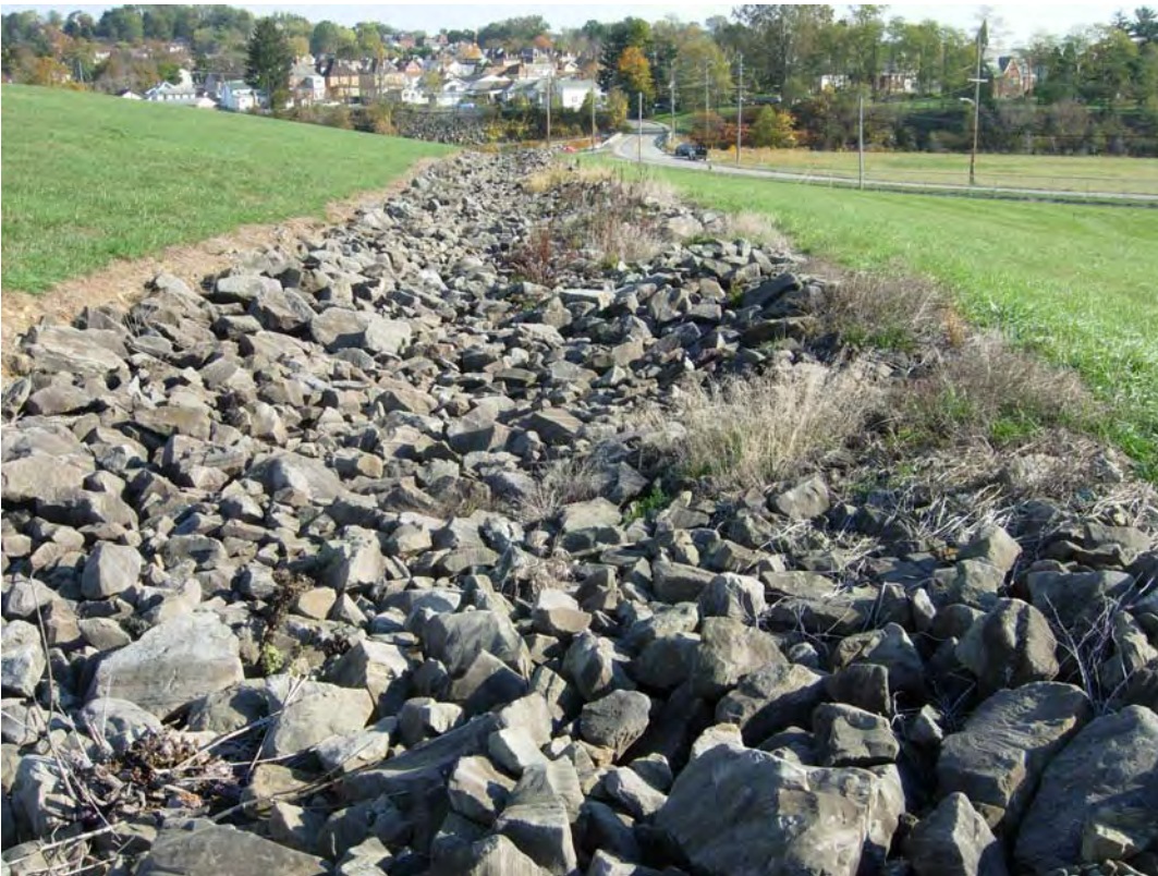
CAN 10/2010. PL-4. Riprap armored diversion ditch.
