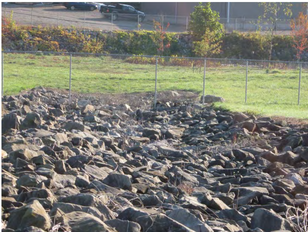
CAN 10/2010. PL-6. Looking down channel of a riprap armored diversion ditch.
