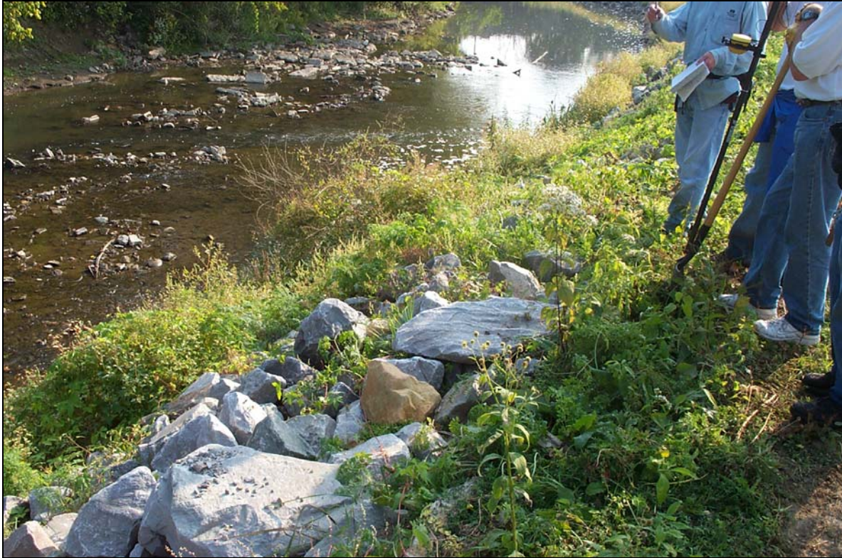
CAN 9/2007. PL-5. Vegetation encroaching on newly installed riprap along Chartiers Creek between perimeter signs P7 and P8.
