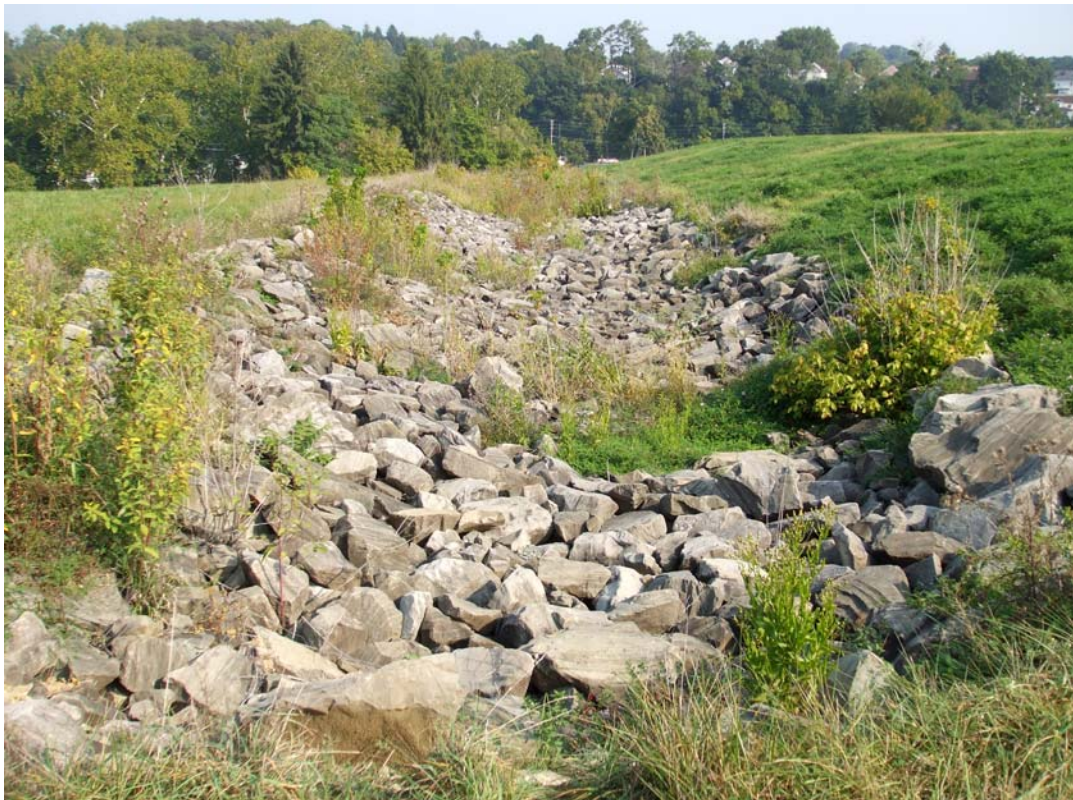
CAN 9/2007. PL-4. Vegetation growing in west diversion channel.
