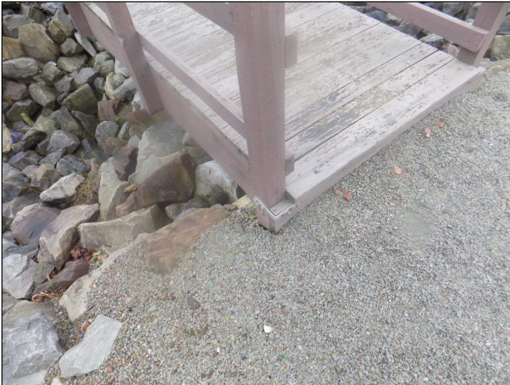
PL-7. Temporary Repair to Pedestrian Footbridge Rail Support
