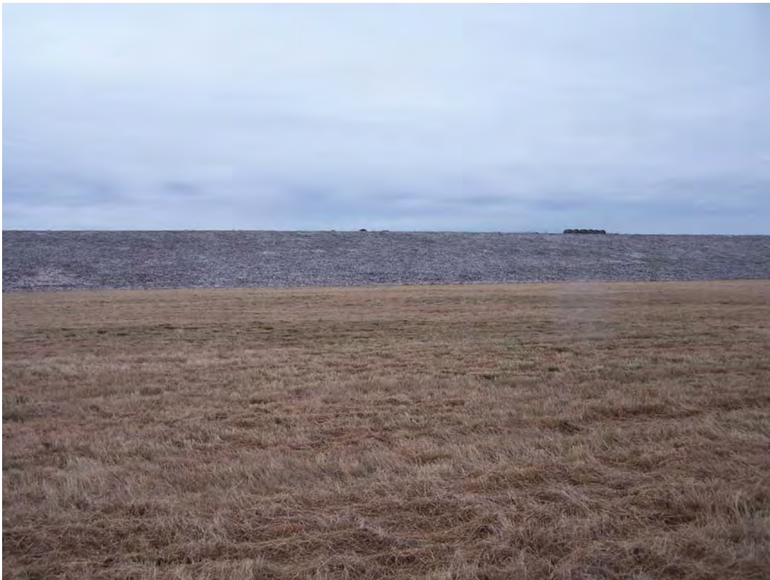
FCT 1/2008. PL-2. Southeast side slope of the disposal cell.
