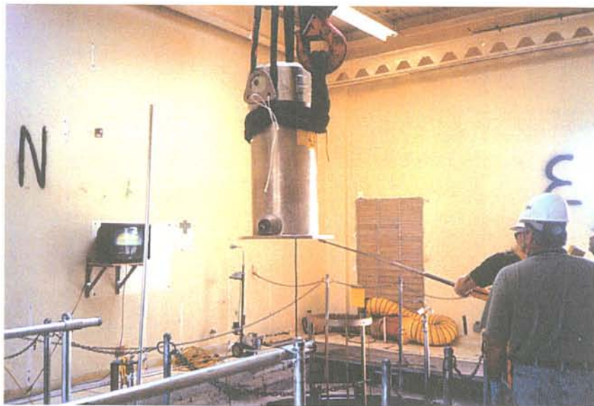
Fig. G-8. Lowering of HTGR/IFM Storage Cask into Dry Pit in Rm. 21/111, 9/19/03
