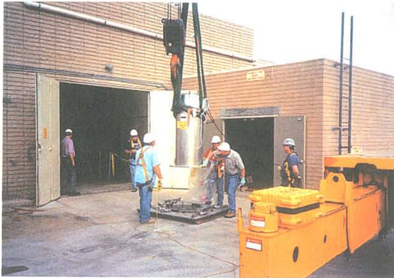
Fig. G-7. Hoist of GA Storage Cask containing HTGR/IFM (note redundant rigging), 9/19/03
