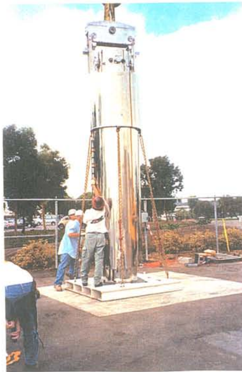
Fig. G-2. NAC-LWT Cask Uprighted/Positioned/ Tied-down to Cask Base Fixture, 9/16/03
