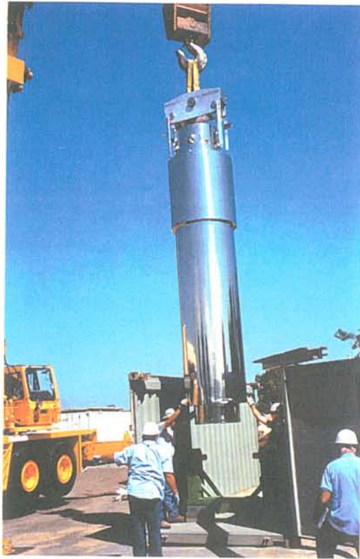
Fig. G-19. Hoist and Translation of Loaded NAC-LWT Cask, 9/20/03
