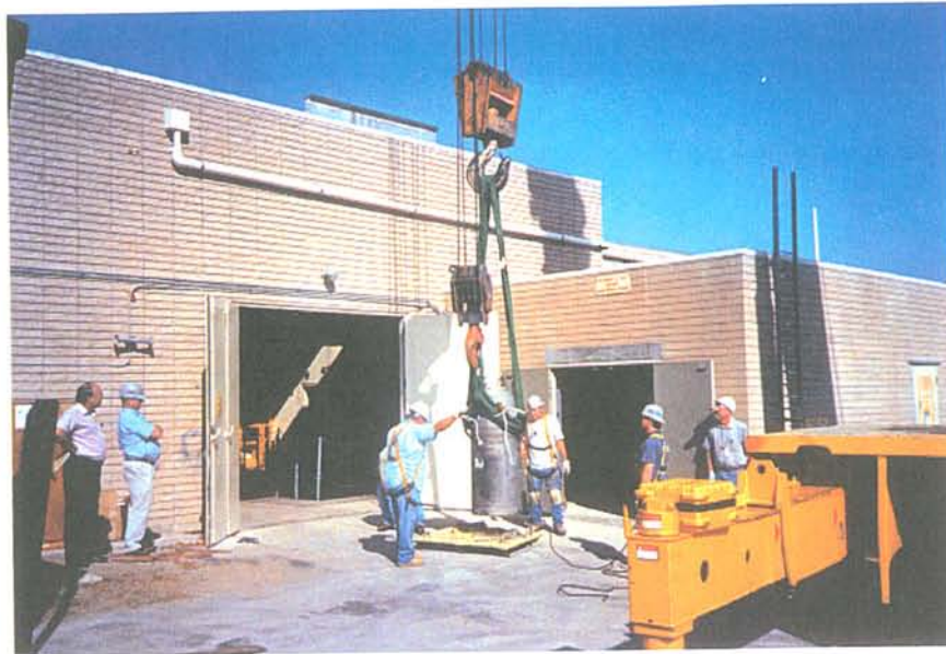
Fig. G-9. Hoist of GA Storage Cask containing RERTR/IFM, (note redundant rigging), 9/19/03
