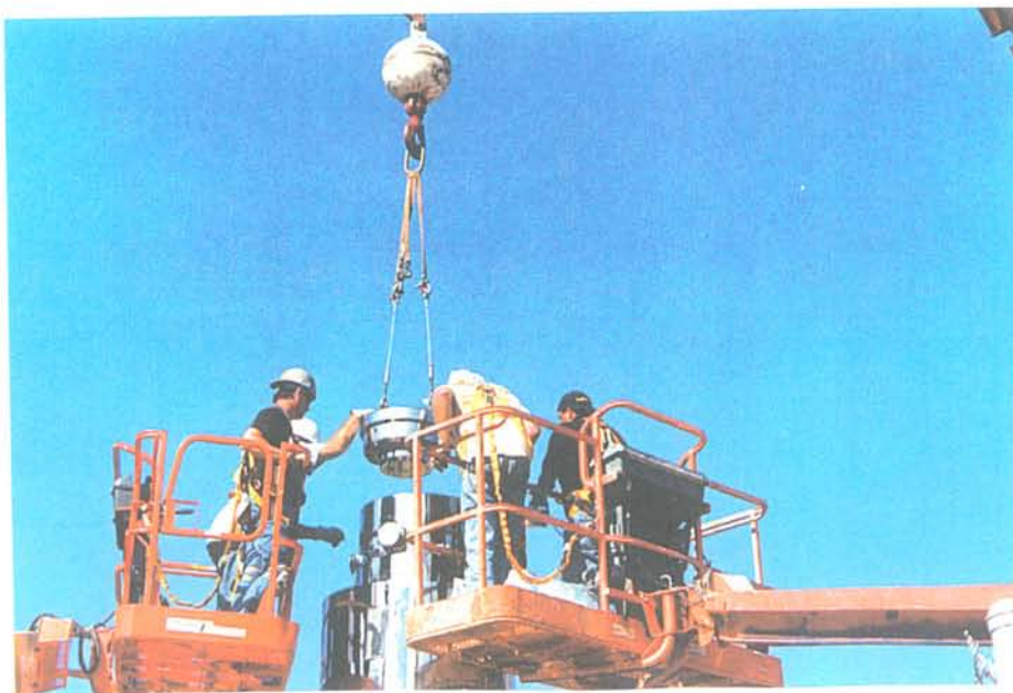
Fig. G-18. Closure Lid Placement on NAC-LWT Cask, 9/20/03
