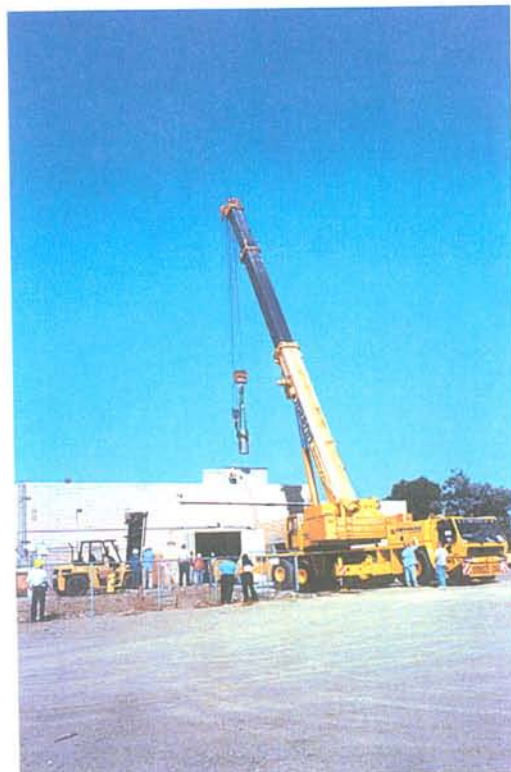
Fig. G-10. Lowering of RERTR/IFM Storage Cask thru Roof Hatch over Rm. 21/111, 9/19/03
