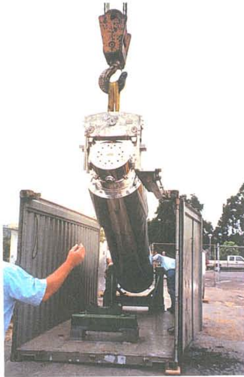
Fig. G-1. Hoist and Removal of NAC-LWT Cask from ISO Shipping Container in GA Bldg. 21 Yard, 9/16/03
