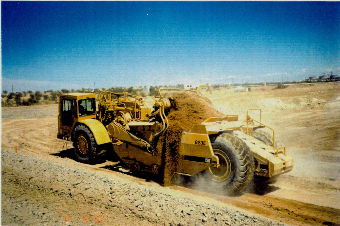
Brine residue being removed from pond
