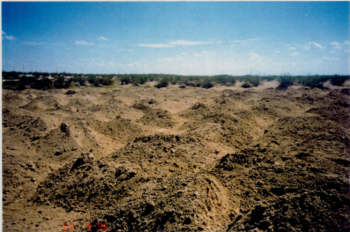
Pond filled with clean material
