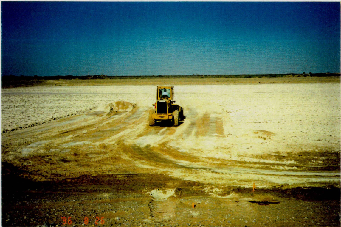
Brine residue being removed from pond
