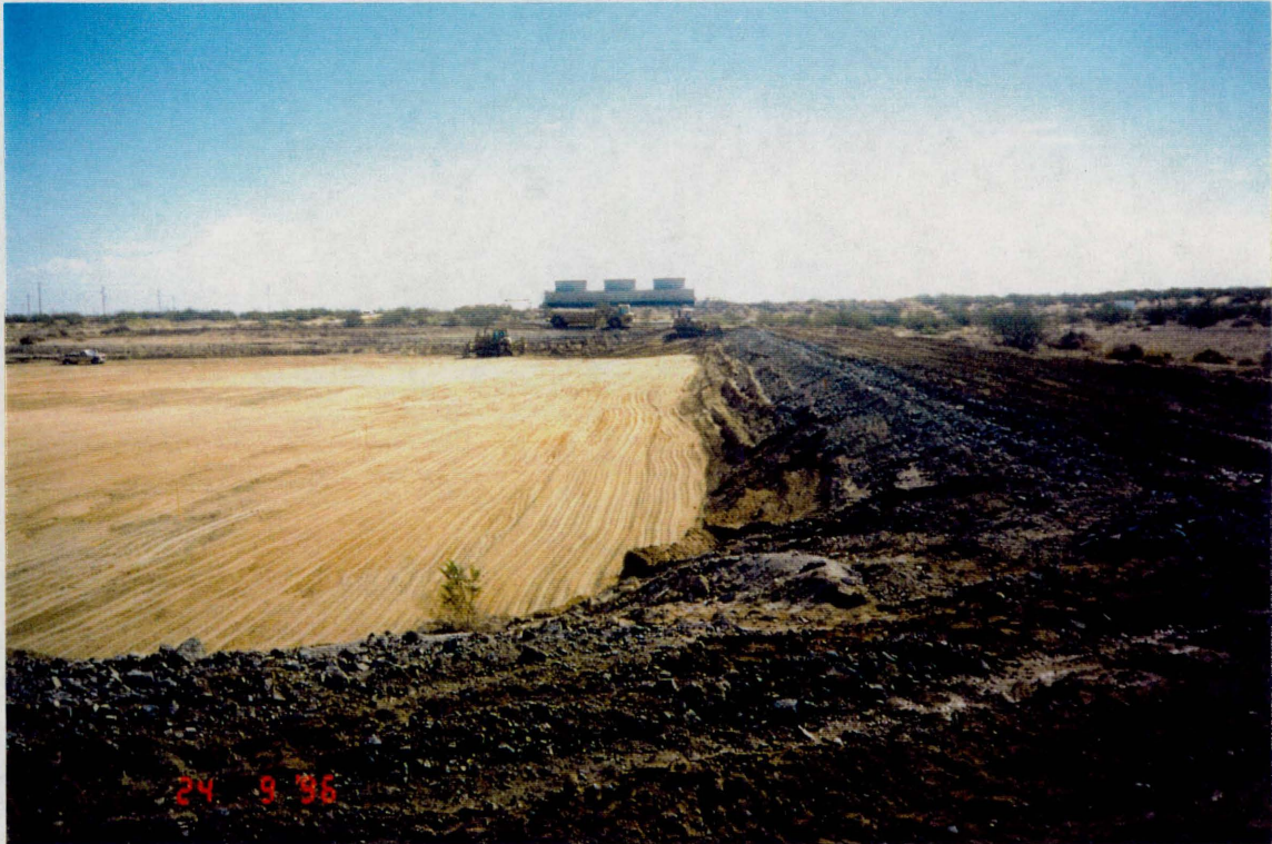
Brine residue removed and berms flattened
