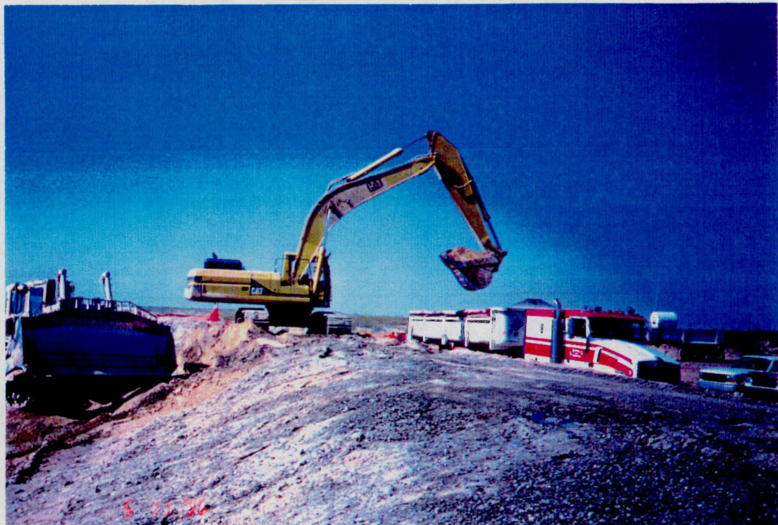
Brine residue being removed from pond
