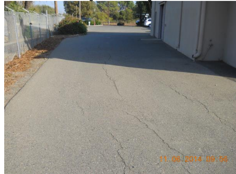
View north over northern portion of Radium/Strontium Treatment Systems Area: Building H-219 to right.
