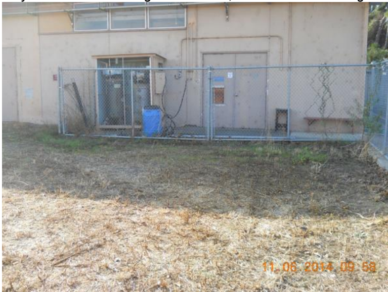
View south over Domestic Septic System 2 area within Radium/Strontium Treatment Systems Area: Building H-218 in background.
