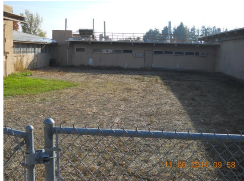
View east over middle portion of Radium/Strontium Treatment Systems Area: Building H-218 to right; Building H-219 to left.
