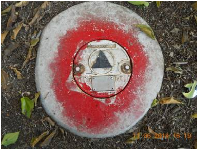
UCD1-071 Wellhead (photo of completed maintenance in Appendix E).
