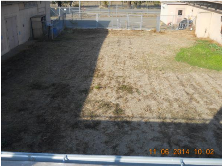
Roof-level view west over middle portion of Radium/Strontium Treatment Systems Area: Building H-219 to right, Building H-218 to left.
