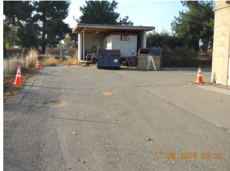
View south over east end of Domestic Septic System 3 leach field: trailer in background.
