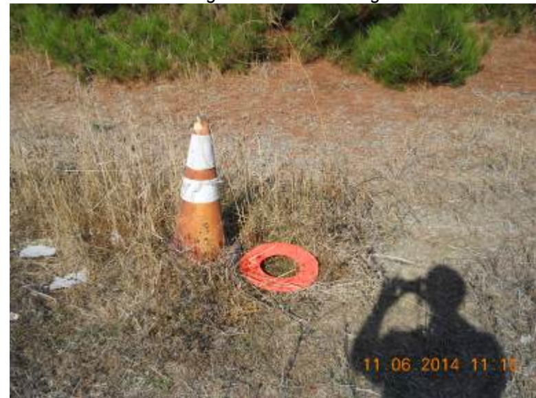
View northwest: Monument 22, within orange ring; Eastern Dog Pens Area trees in background.
