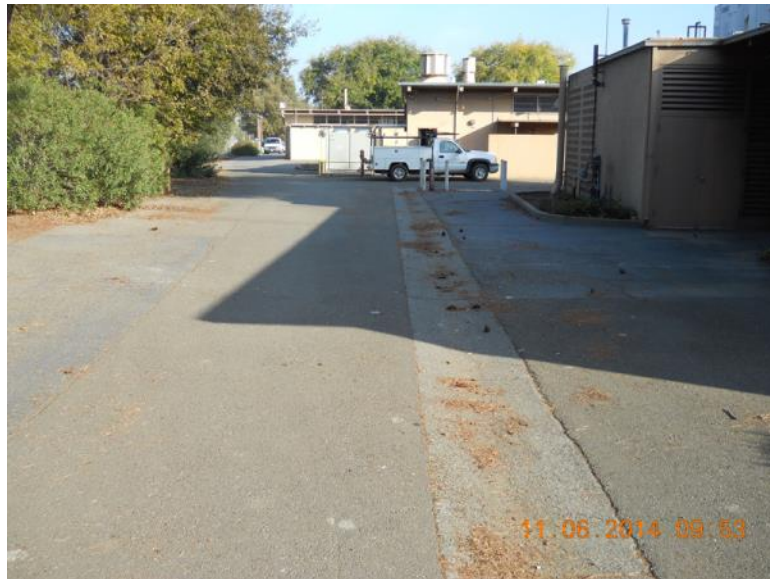
View north over southern portion of Radium/Strontium Treatment Systems Area: Building H-215 to right; Buildings H-218 and H-219 in background.
