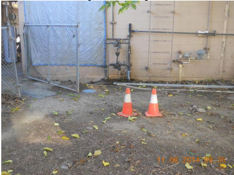
View east over Domestic Septic System 4 septic tank location: Building H-216 in background.
