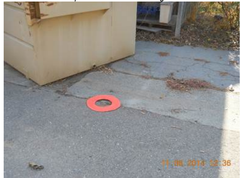
View southeast: Monument 24, within orange ring on edge of concrete swale—waste bin and trailer shed behind; rose planter in right of background.
