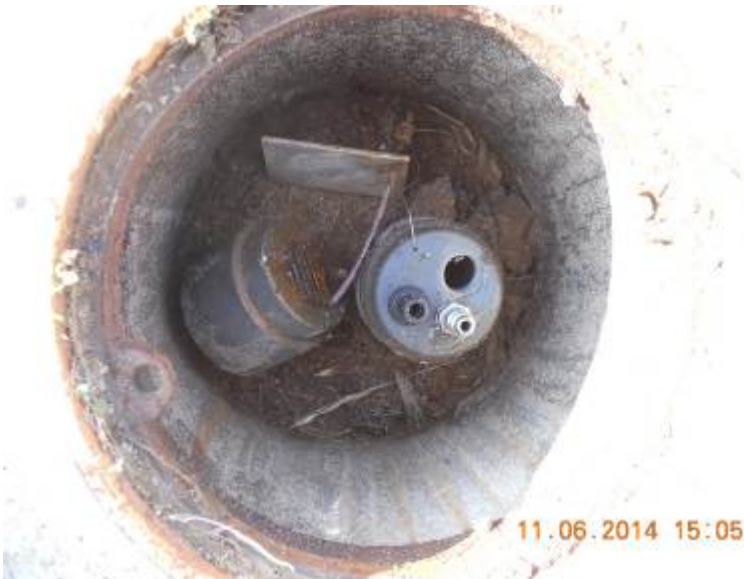
UCD1-069 Interior (photo of completed maintenance in Appendix E).
