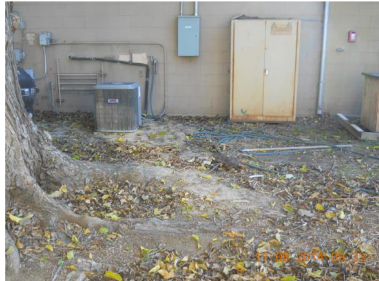
View east: Building H-216 in background, standing south/right of tree.
