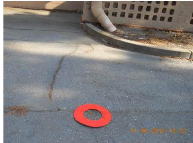
View east: Monument 5, within orange ring; Building H215 in background.
