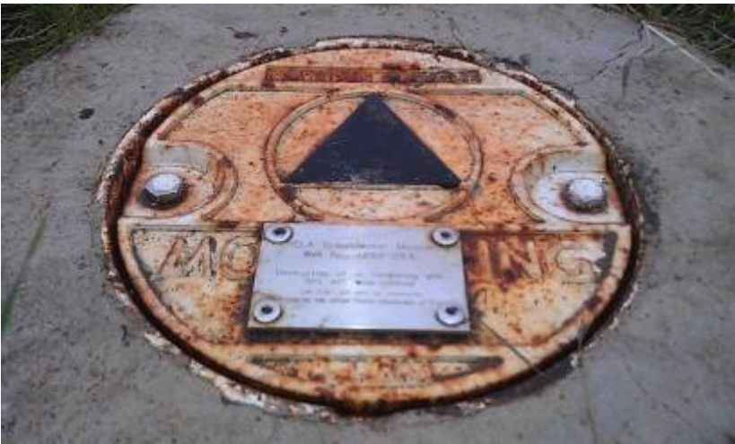
UCD1-068: threads cleaned, bolts tightened, and lid secured.
