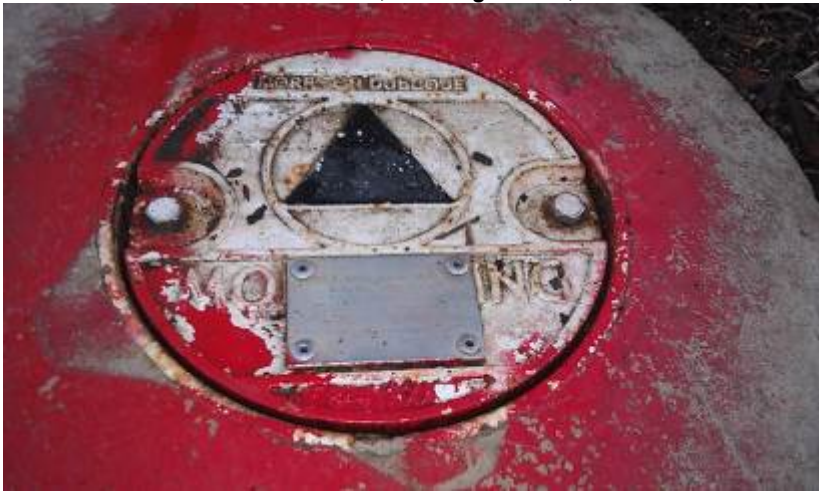
UCD1-071: threads cleaned, bolts tightened, and lid secured.
