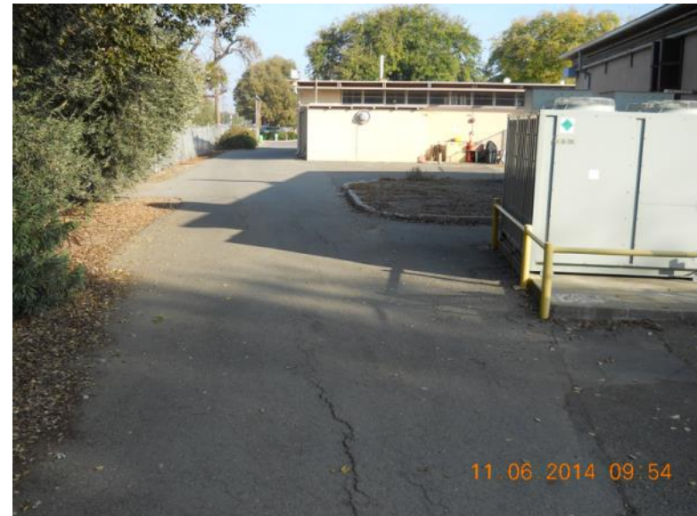
View north over middle portion of Radium/Strontium Treatment Systems Area: Building H-218 at the upper right-hand corner, Building H-219 in background.
