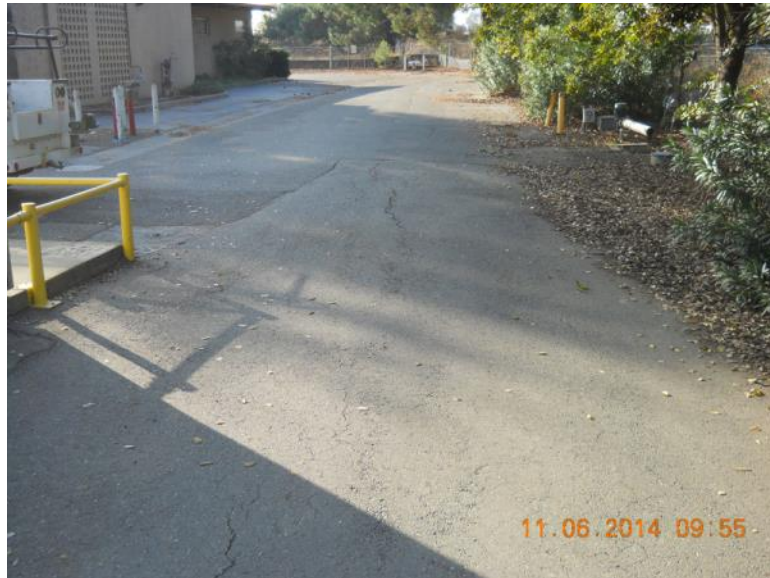
View south over southern portion of Radium/Strontium Treatment Systems Area: Building H-215 to left.
