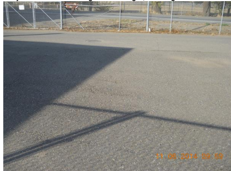
View west over middle-west portion of Radium/Strontium Treatment Systems Area, west perimeter fence, and Old Davis Road.
