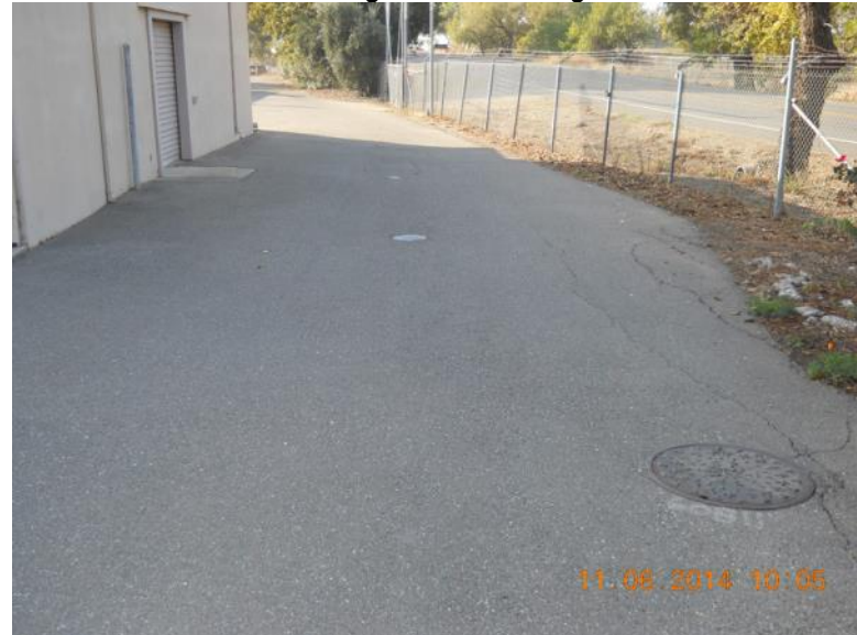
View south over northern portion of Radium/Strontium Treatment Systems Area.
