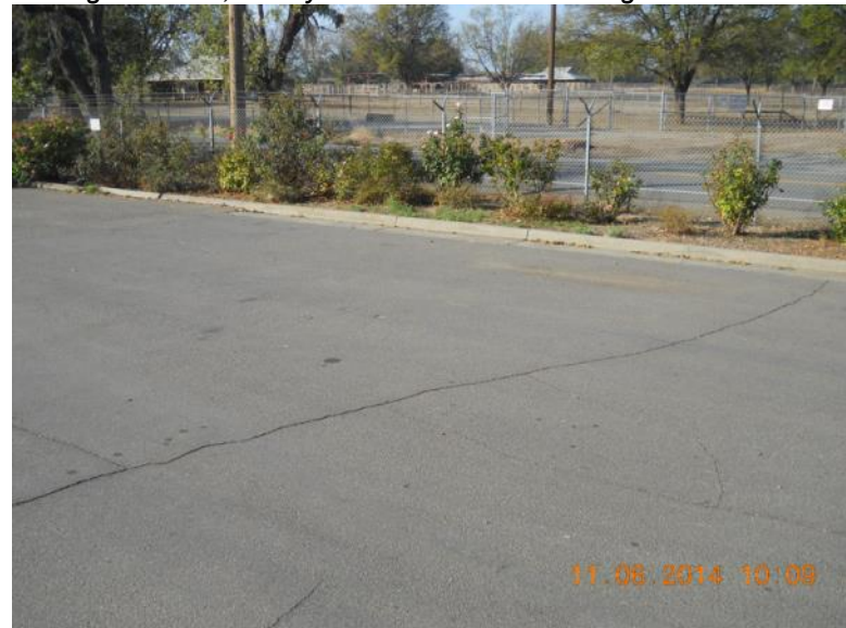
View southwest over Dry Wells A-E Area: Old Davis Road in background.
