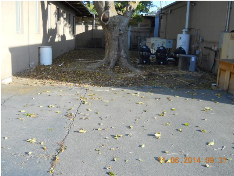
View north over septic tank part of Domestic Septic System 3 Area: Building H-215 to left, Building H-216 to right; Domestic Septic System 4 Area in background.
