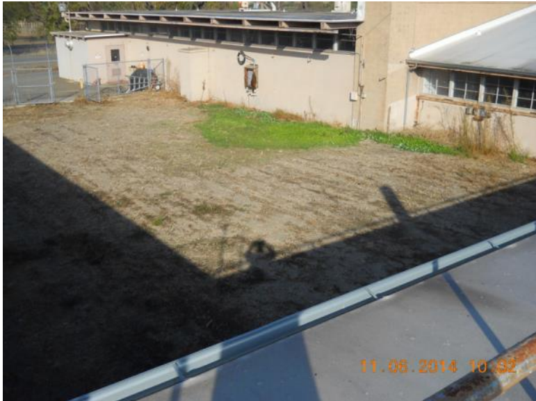
Roof-level view northwest over middle portion of Radium/Strontium Treatment Systems Area: Building H-219 in background.
