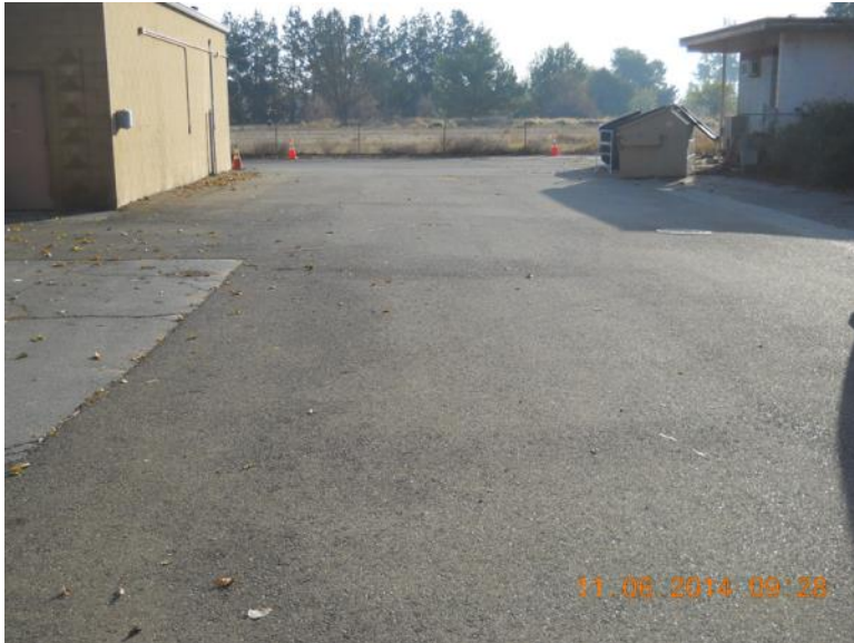
View east over former leach field part of Domestic Septic System 3 Area: Building H-216 to left; storage unit to right; Western Dog Pens Area in background.
