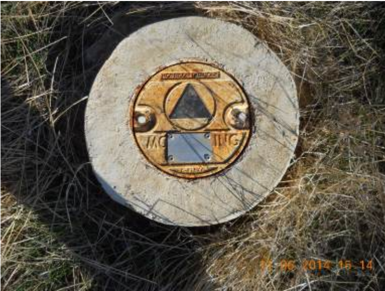
UCD1-068 Wellhead (photo of completed maintenance in Appendix E).
