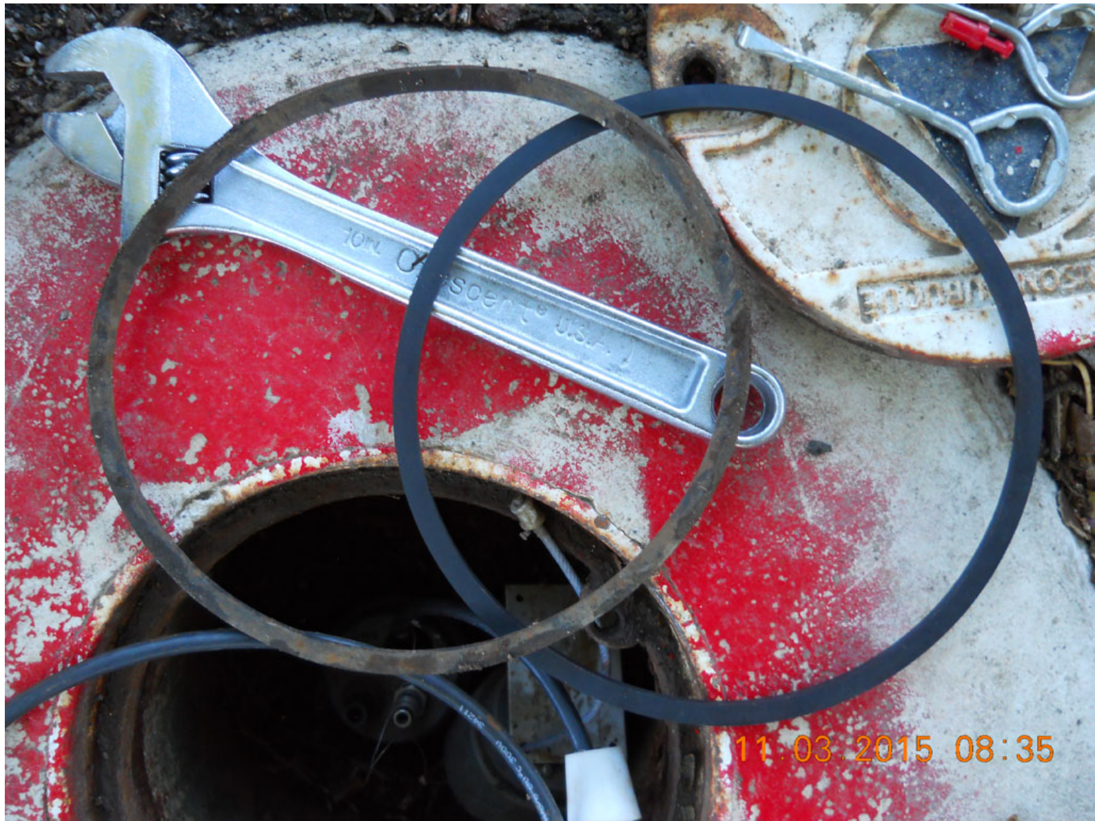
UCD1-071: vault lid gasket replacement.
