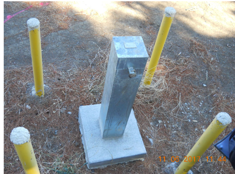
Well UCD1-070 after concrete apron replacement (photo No. 3443).
