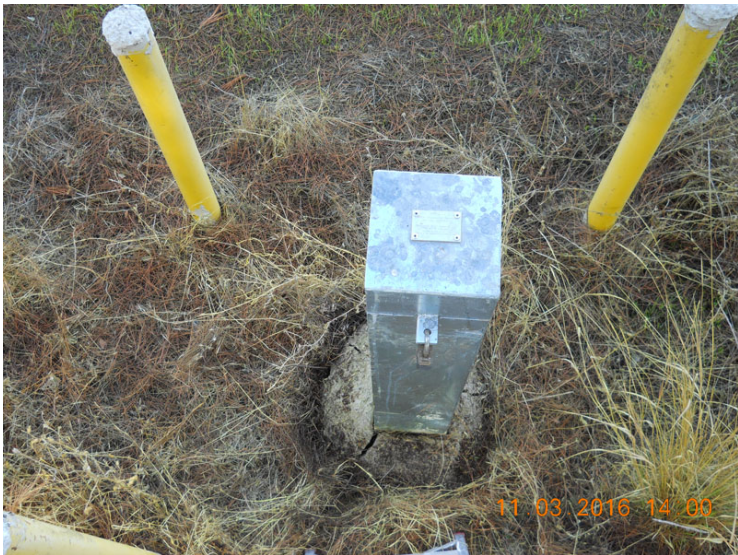
Well UCD1-070 before concrete apron replacement (photo No. 3222 from 2016 inspection report).
