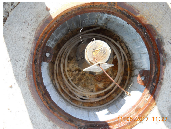
Well UCD1-021 vault interior after replacement (photo No. 3440).
