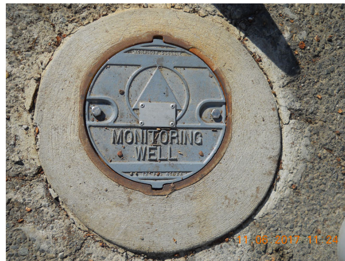
Well UCD1-021 wellhead after vault replacement (photo No. 3437).
