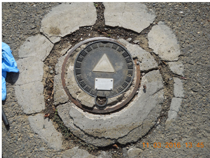
Well UCD1-021 wellhead before vault replacement (photo No. 3218 from 2016 inspection report).
