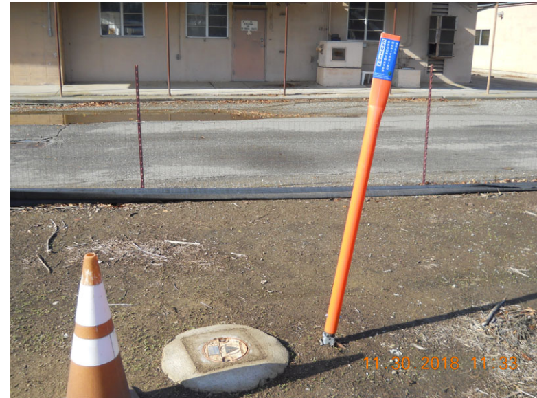
Well UCD1-072 and delineator with decal.
