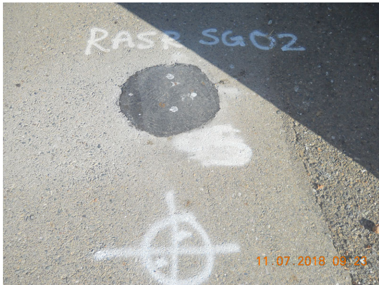
Radium/Strontium Treatment Systems Area: Decommissioned soil gas well RASRSG-02 (photo No. 3612).
