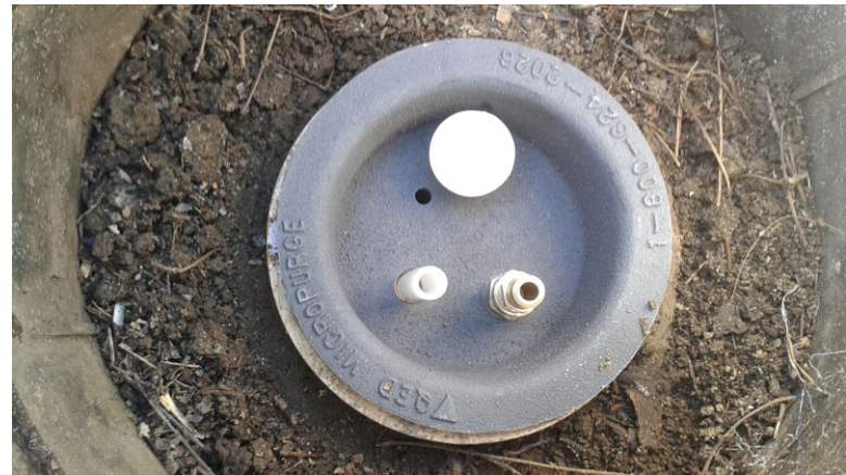
Well UCD1-023 vault after pump replacement.
