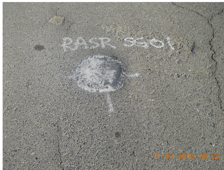
Radium/Strontium Treatment Systems Area: Decommissioned soil gas well RASRSG-01 (photo No. 3611).
