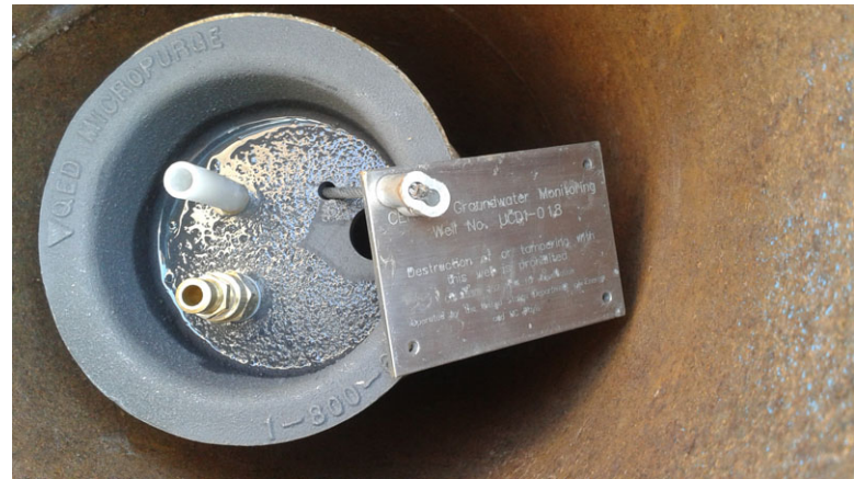
Well UCD1-018 vault after pump replacement.
