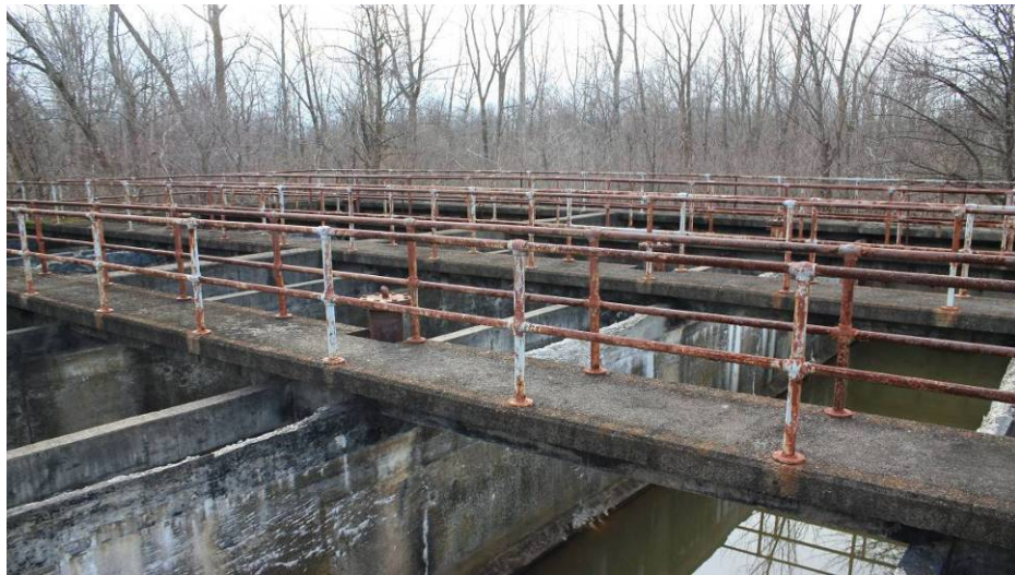
Figure 5-13. VP-X: IMHOFF Tank
