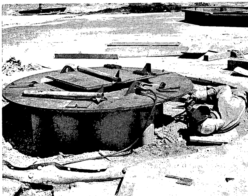
Figure 12 Welding Cover Plate to Casing - Sta. UC-3
