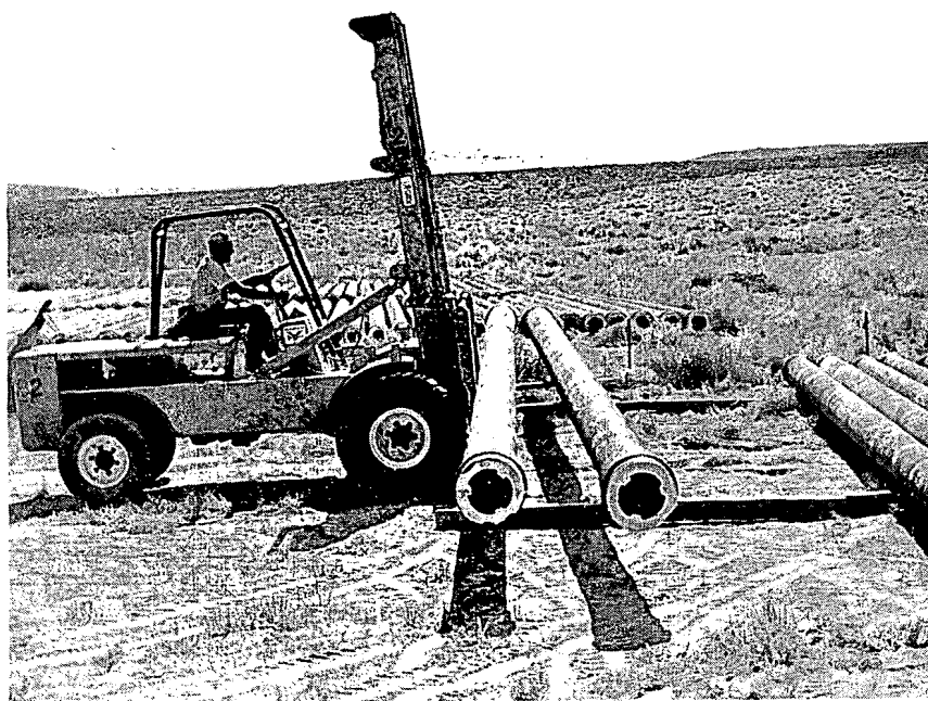
Figure 16 Moving Drill Pipe into the Pipe Yard
