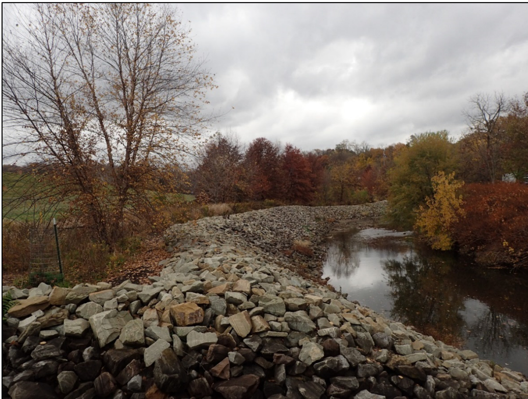
PL-10. Riprap-Armored Streambank
