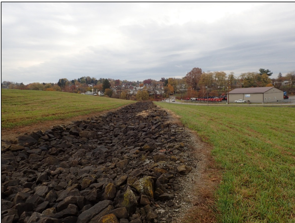
PL-8. Riprap-Armored Diversion Channel
