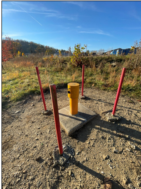
PL-3. Repaired Well Pad at Monitoring Well 0424
