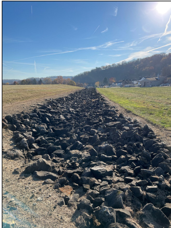
PL-5. Riprap-Armored Diversion Channel
