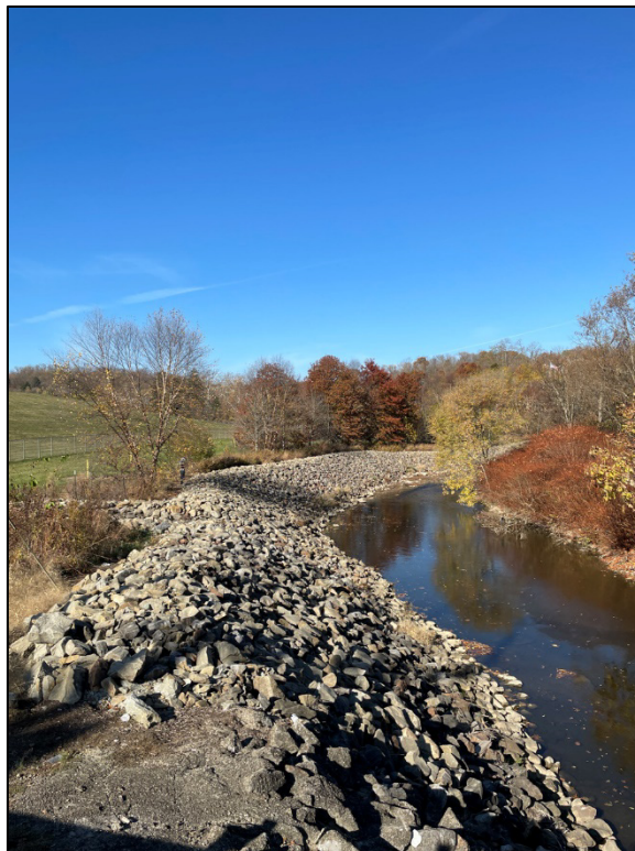
PL-6. Riprap-Armored Streambank
