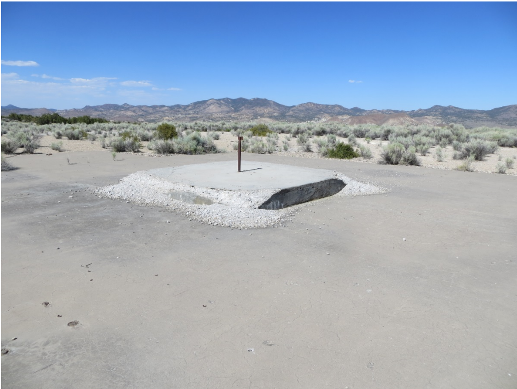
Figure A-2. Concrete Cap that Covers the UC-4 Emplacement Borehole
