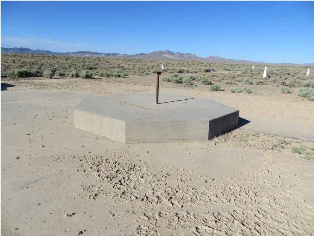
Figure A-1. Concrete Cap that Covers the UC-3 Emplacement Borehole
