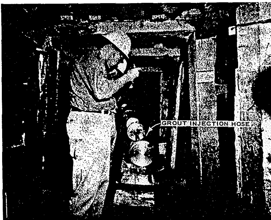
Figure 3.7 Instrument array immediately prior to emplacement in hole PM-5. Note grout injection hose near end of the array. (FCWT DASA 160-70-FTS-63).
