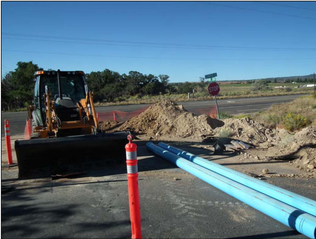
PL-25. Utilities Construction, Looking South on 1075 East and Center Street
