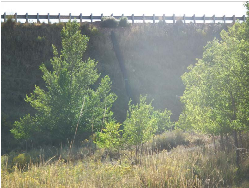
PL-26. U.S. Highway 191 Embankment
