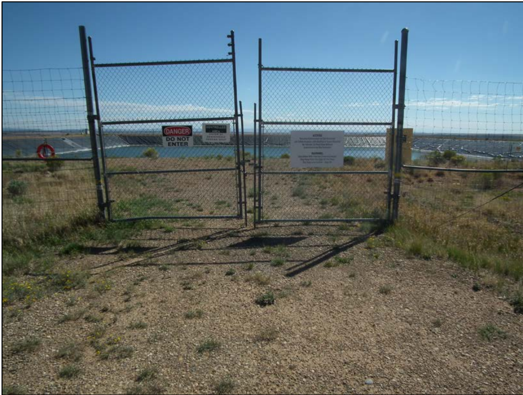
PL-13. Pond 4 Entry Gate
