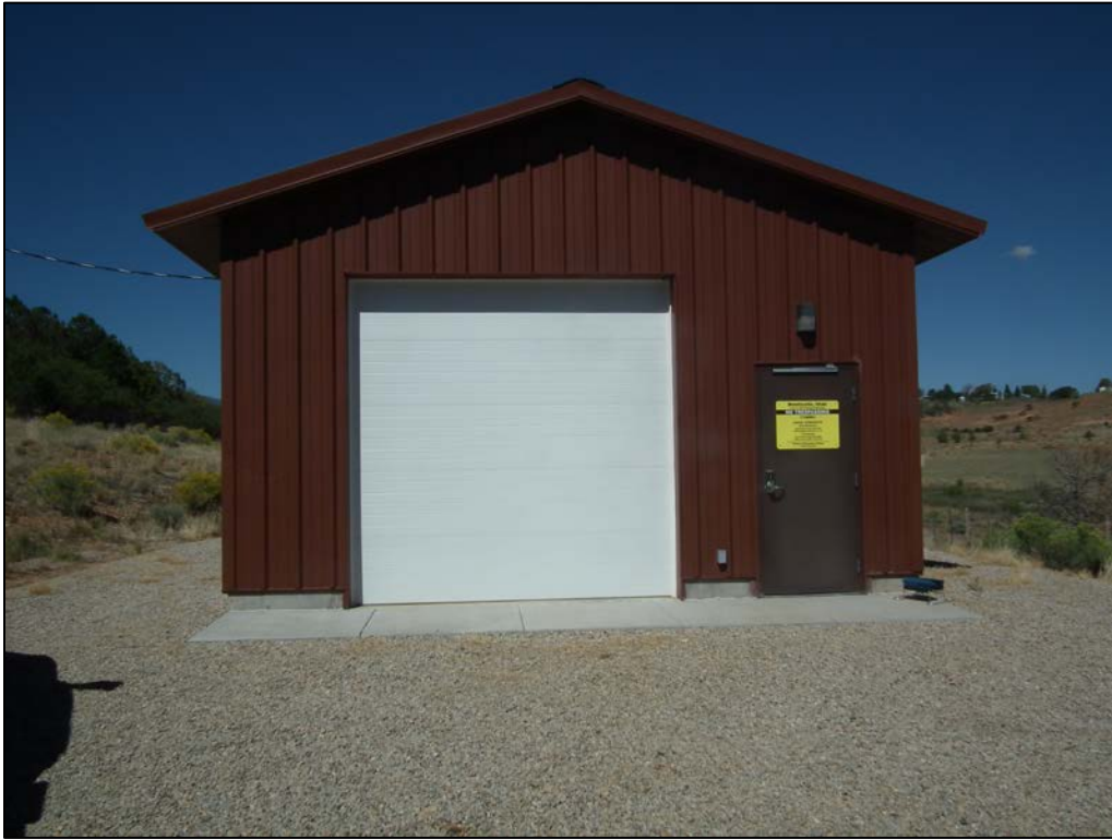
PL-28. Transfer Building, Looking West
