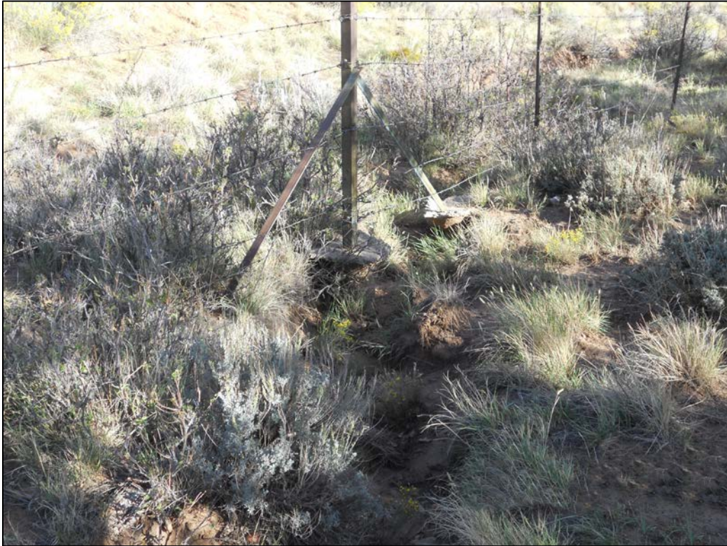
PL-5. Repaired Gap in Northwest Fence Line
