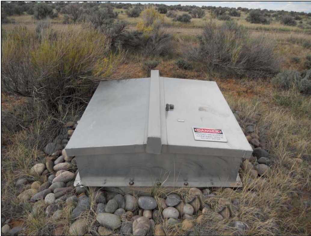
PL-17. Looking North from Manhole 1
