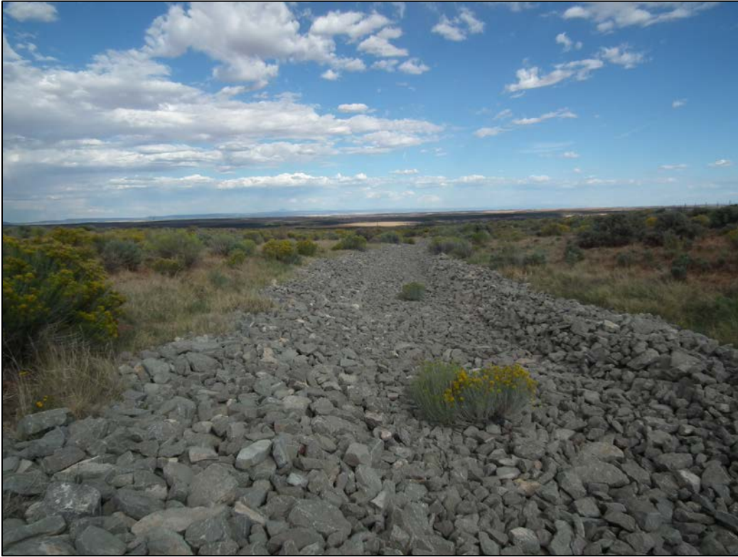
PL-11. West Drainage Channel, Looking North
