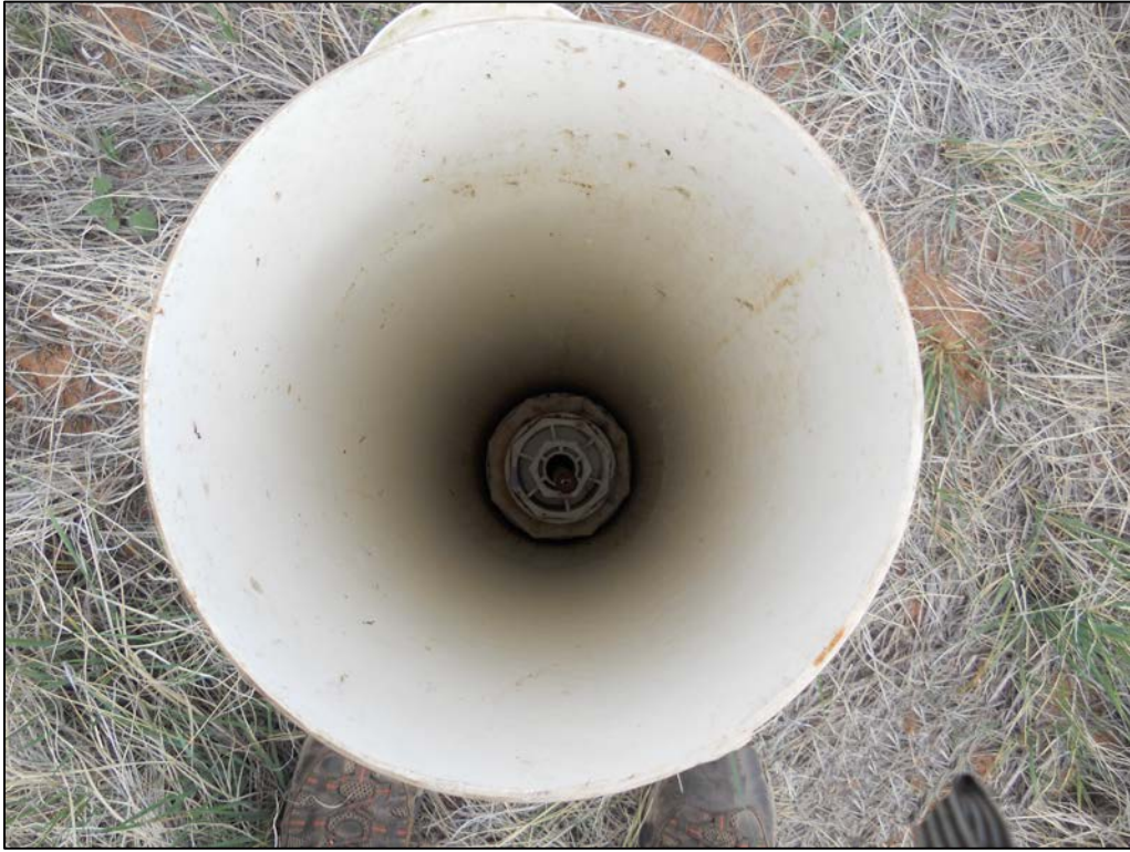
PL-19. Looking at Interior of Settlement Plate A
