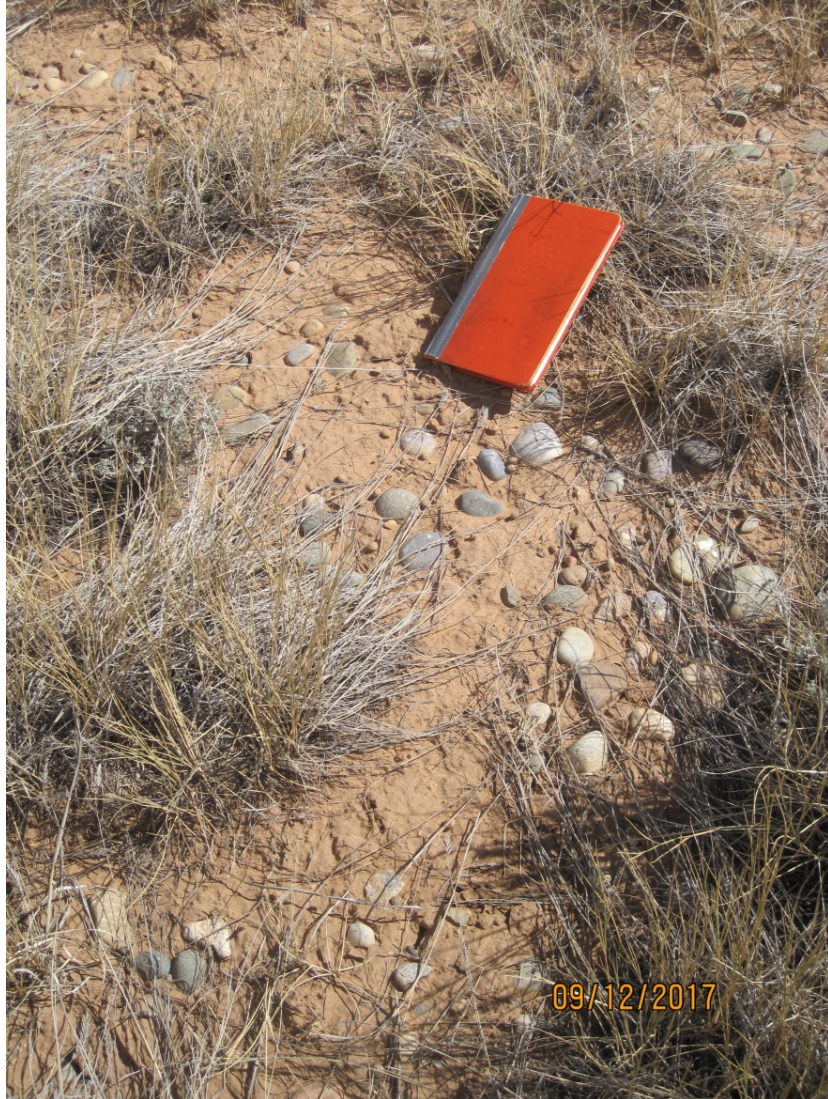
Figure No. 6, Top slope cover, soil/rock matrix and vegetation, (2017 photo)
