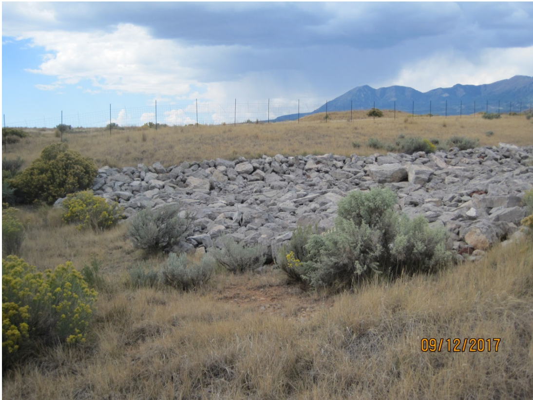
Figure No. 7, Outfall, South diversion ditch (2017 photo)
