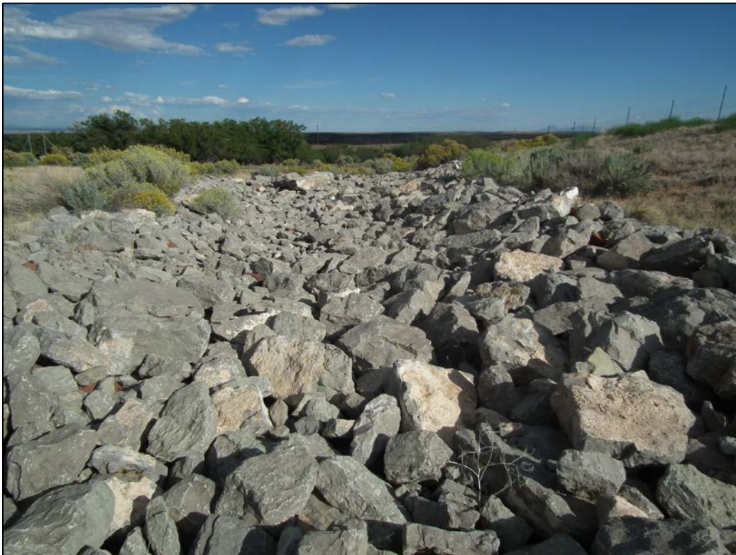
PL-10. South Drainage Channel, Looking East
