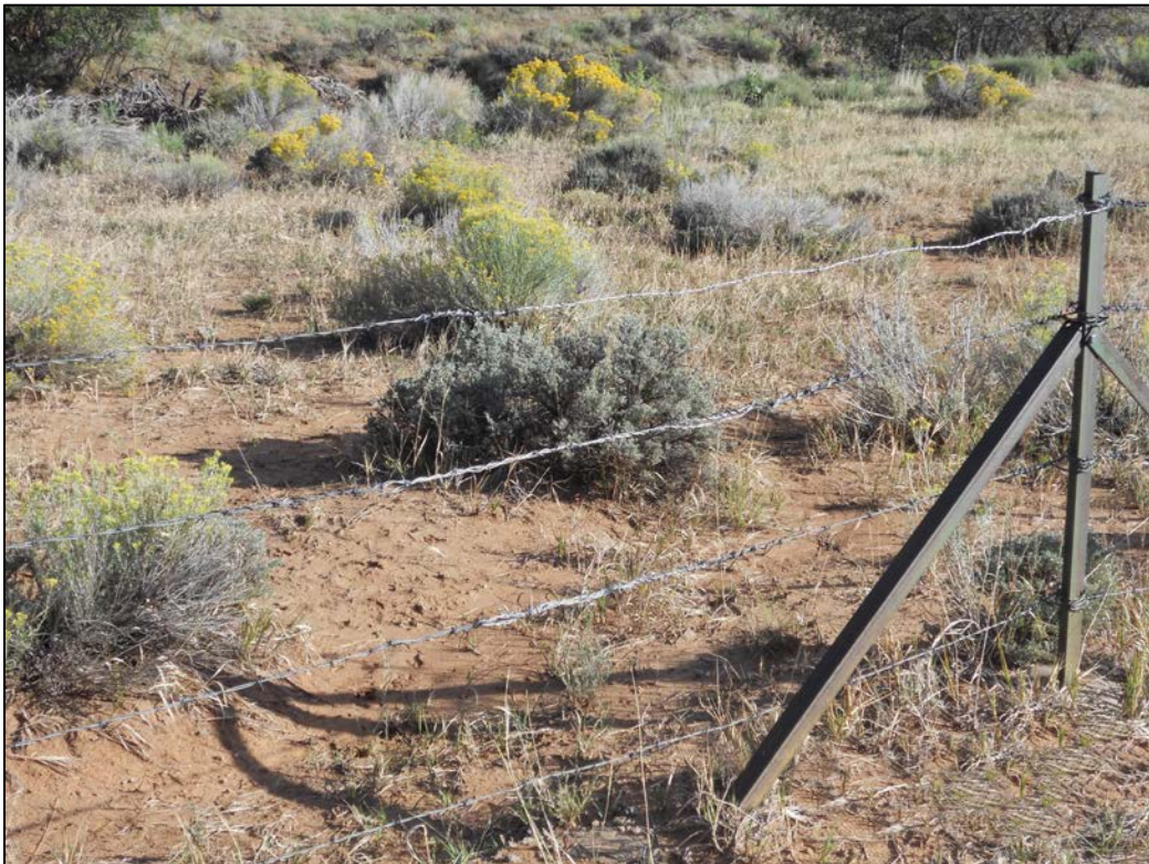
PL-6. Northwest Fence Repaired from Last Year
