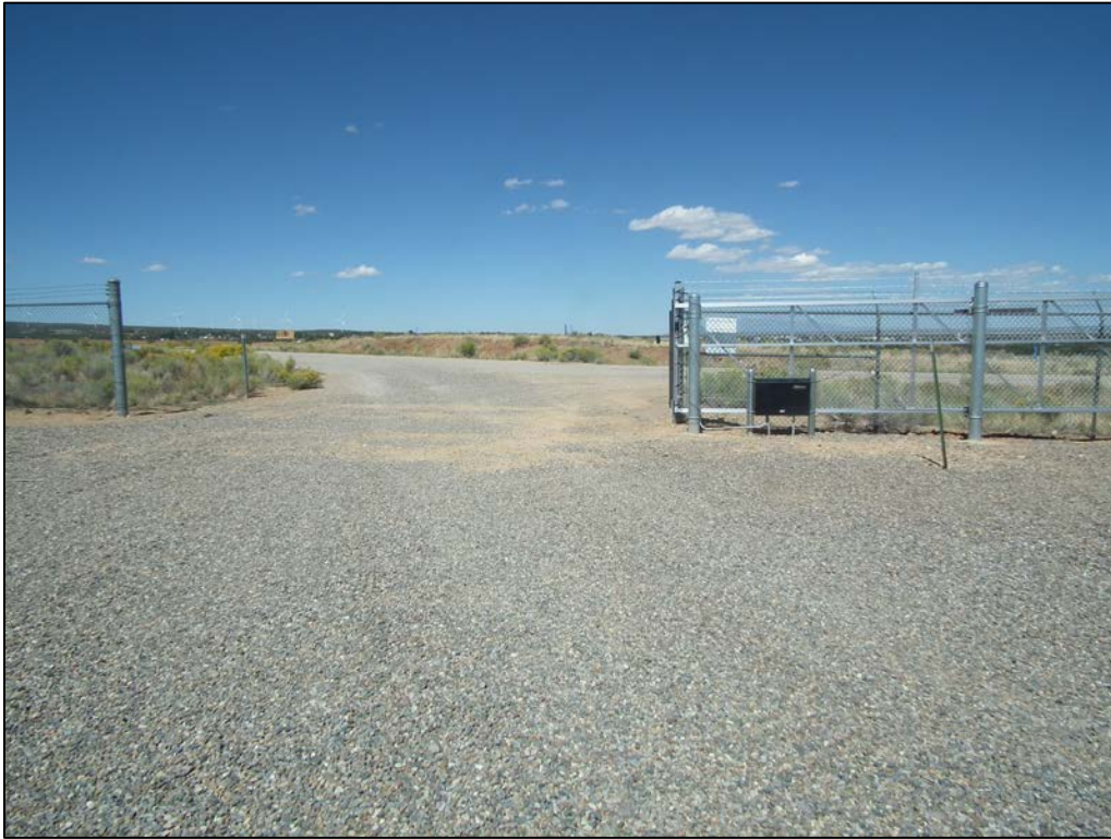
PL-2. New Electric Gate to the Administrative Building
