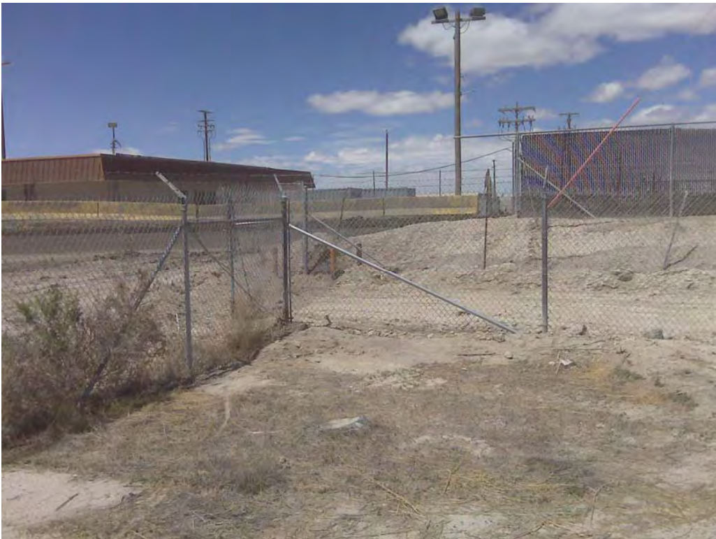
SLC 4/2008. PL-2. Repaired fence and uncovered boundary monument BM-1.
