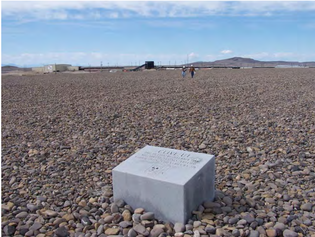
SLC 4/2008. PL-3. Site marker SMK-2 on the disposal cell top.
