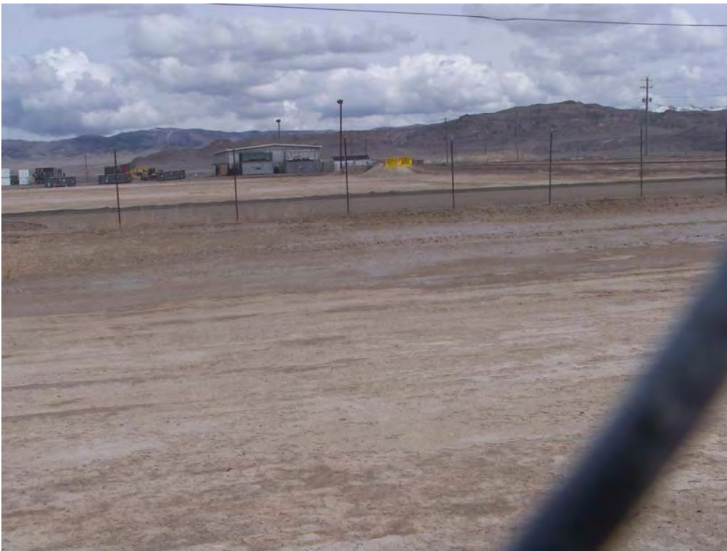
SLC 4/2008. PL-6. Area flooded in June 2007 and repaired berm east of the cell.
