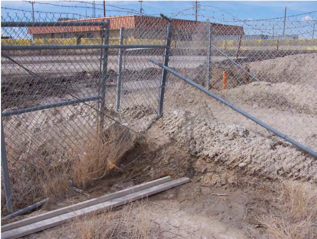
SLC 4/2008. PL-1. Fence damage and buried boundary monument BM-1.
