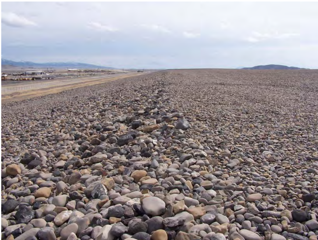
SLC 4/2008. PL-4. East side slope and top of the disposal cell.
