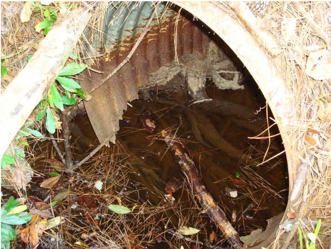
Photo A-1 Culvert with Corrosion of the Base
