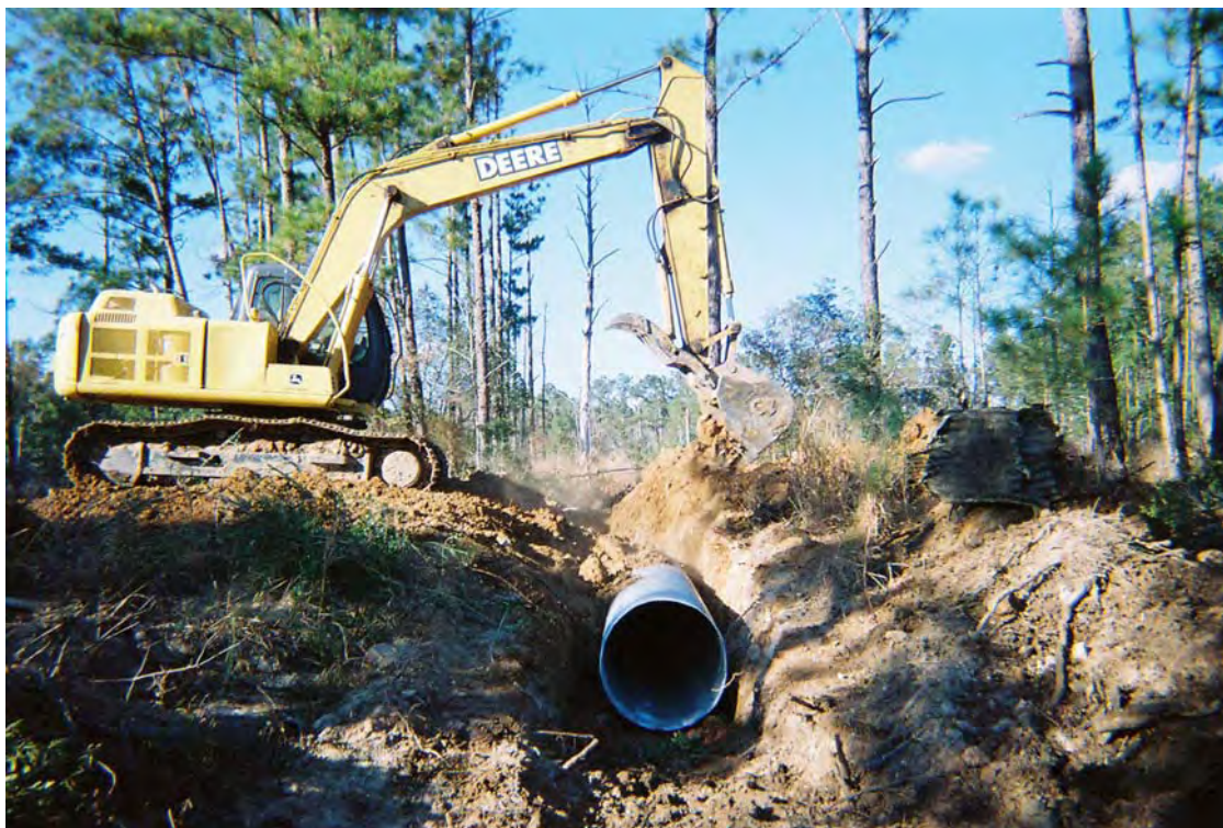
Photo A-3. Installation of Culvert Between North and South Ponds
