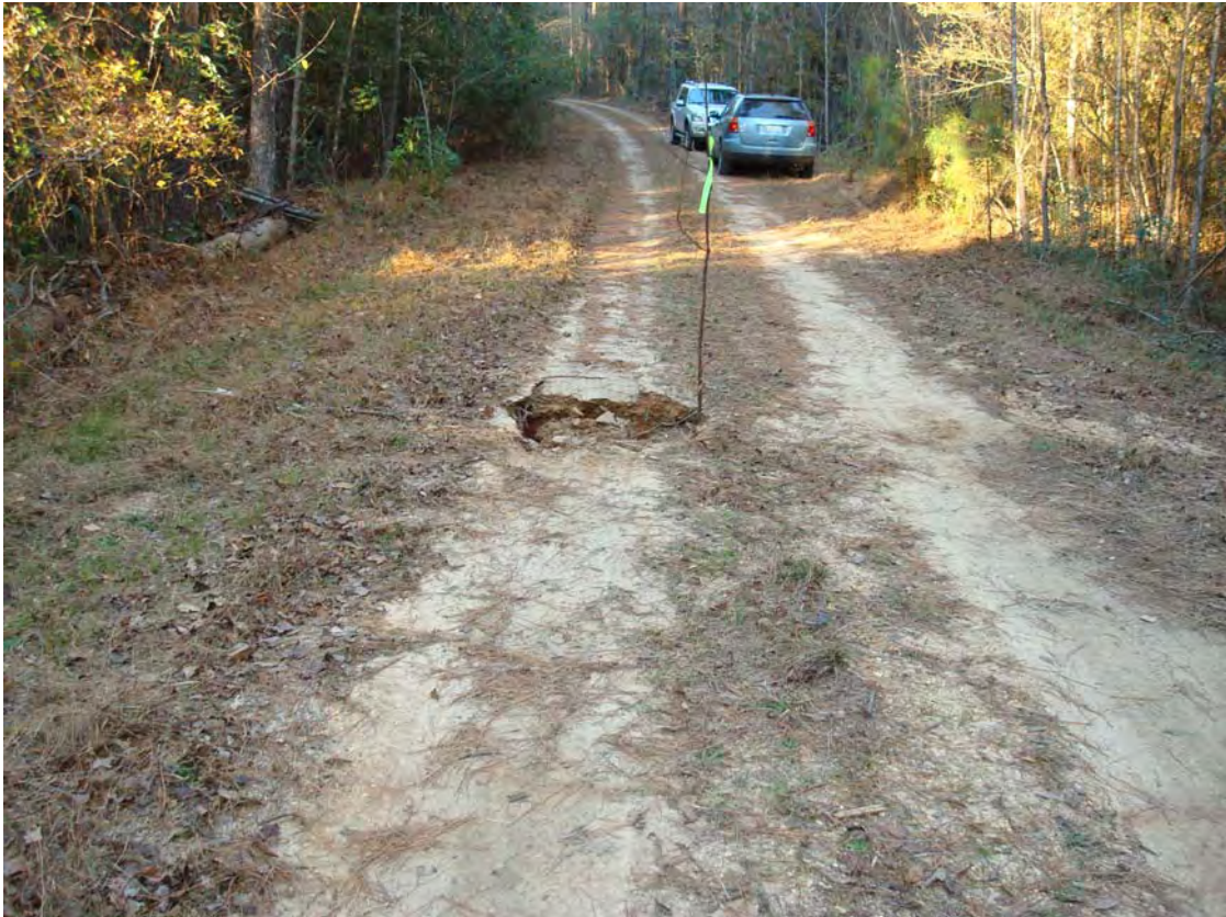
Photo A-2. Sinkhole in Road Caused by Culvert Failure
