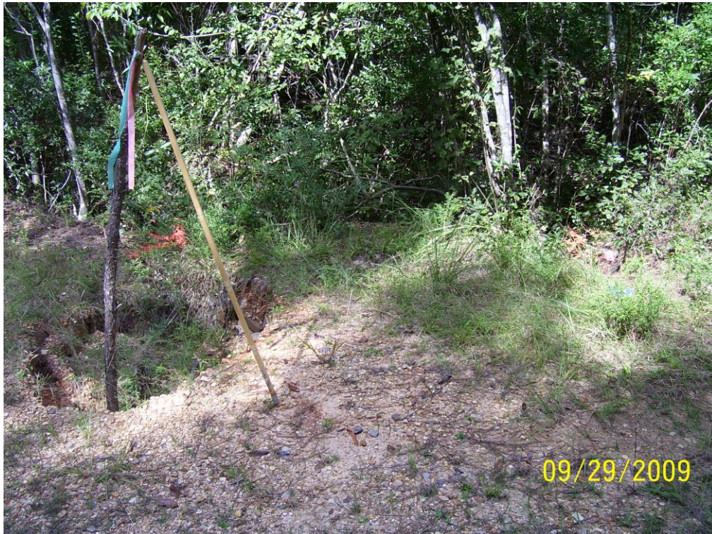
Photo A-3. Sink Hole in Main Road SW Due to Culvert Invert Failure at Location C031
