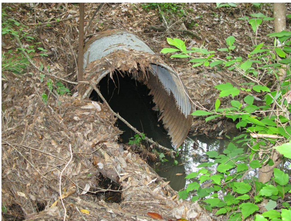
Photo A-2. Typical Culvert Invert Failure
