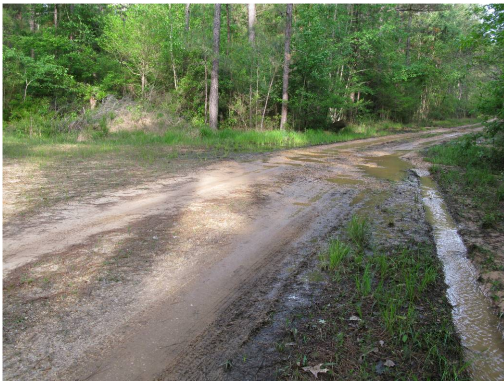
Photo A-1. Water Damage of Main Road NE Caused by a Blocked Culvert Located on the Main Road NE at the Intersection with Northridge Road
