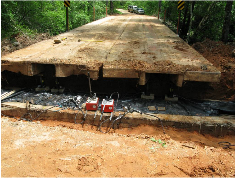
Image A-9. West end of flatcar bridge raised on hydraulic jacks that sit on cribbing.
