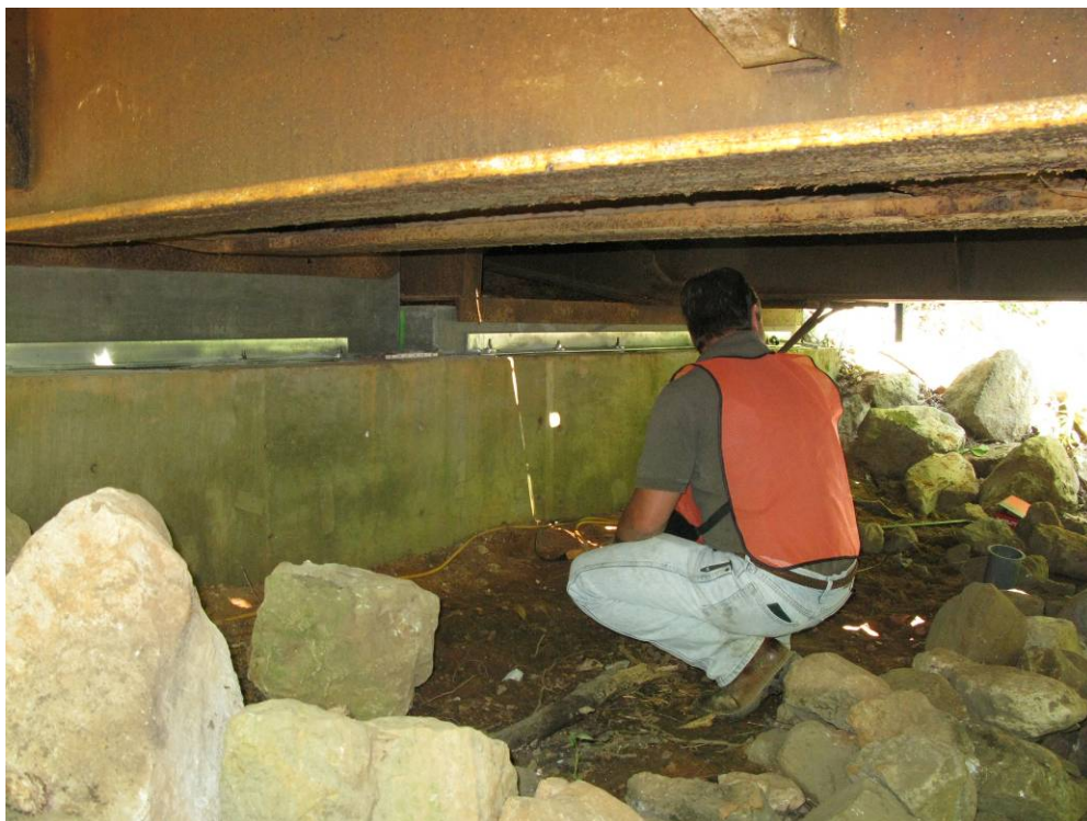
Image A-12. Re-inspection of flatcar bridge after the new concrete head caps are in place and secured by stainless steel angles.
