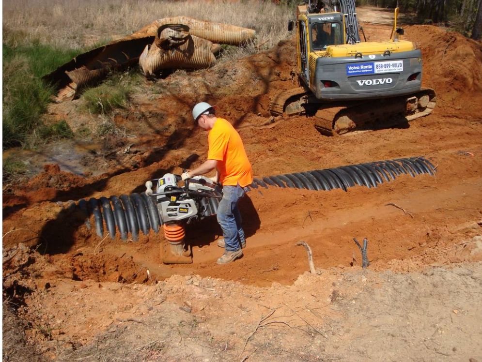
Image A-7. Compacting backfill.
