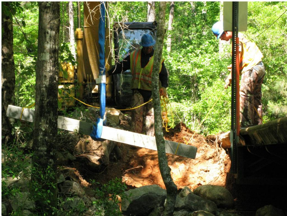
Image A-11. Installation of a new concrete head cap under the west end of the flatcar bridge.
