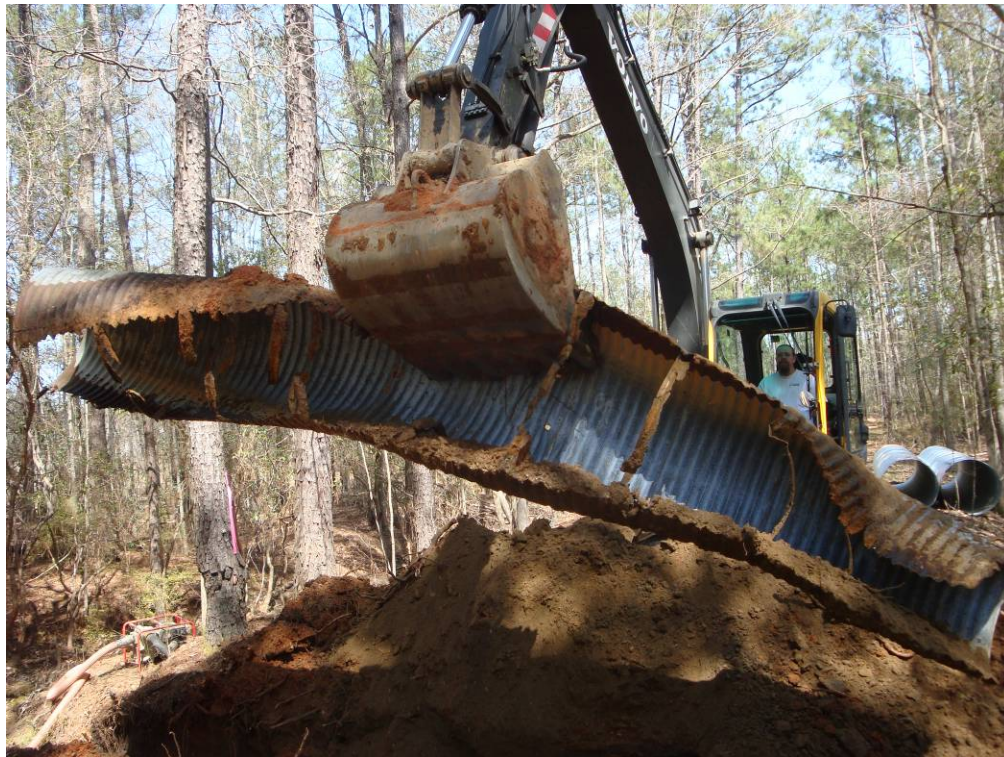
Image A-5. Removal of an old culvert.
