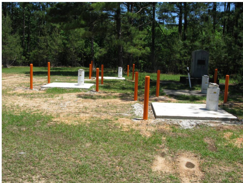
Image A-2. Four ground zero wells, orange bollards, and new concrete well pads are shown. The wells reside inside the white protective casing. The monument (ground zero) is in the background, to the right.
