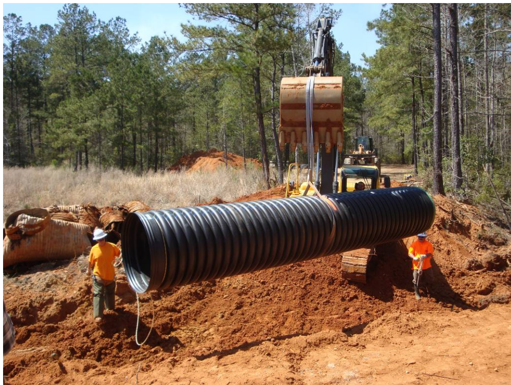
Image A-6. Installation of a new plastic culvert on Beaver Pond Road. Most new culverts that were installed are galvanized steel.
