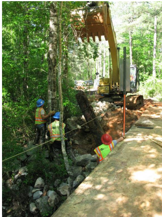
Image A-10. Removing wood head cap from west end of the flatcar bridge.
