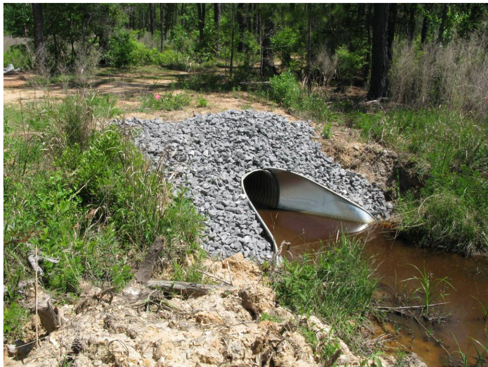
Image A-8. Finished end of a new culvert.
