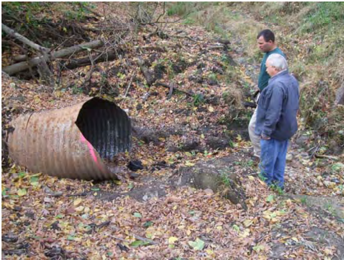
Photo 5. Culvert under Highway 94.
