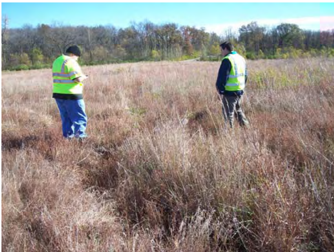
Photo 24. Erosion areas north of the disposal cell, showing vegetative growth.
