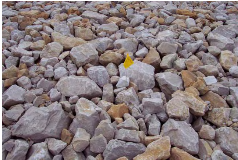
Photo 3. Cell cover rock test plot TP2; north edge north facet (2003 Inspection).
