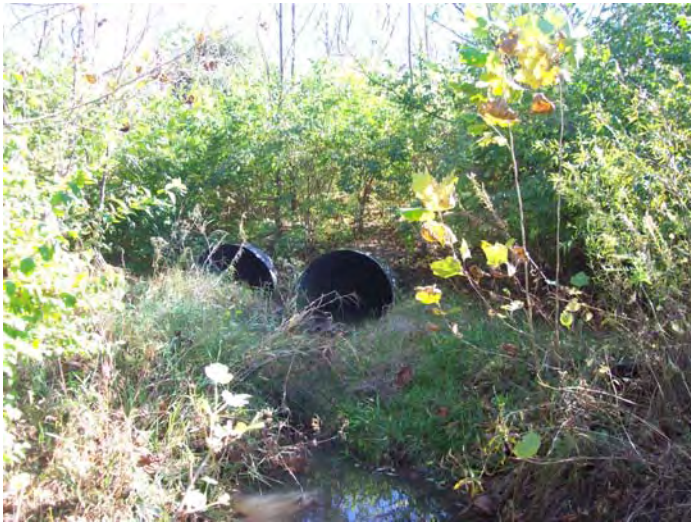
Photo 4. Highway D culverts outlet.
