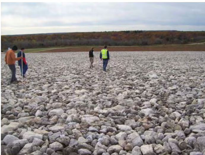
Photo 6. Disposal cell inspection looking south.
