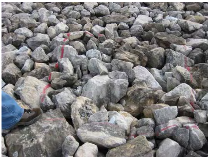
Photo 21. Cell cover test plot TP5; located on lower west side.
