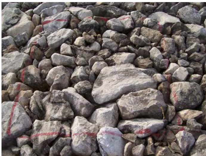
Photo 9. Cell cover test plot TP1; north edge of north facet.
