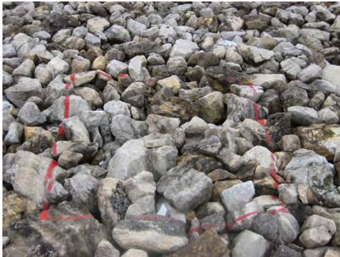
Photo 10. Cell cover rock test plot TP5; located on lower west side (2009 Inspection).
