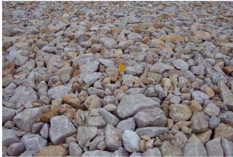
Photo 1. Cell cover rock test plot TP1; north edge north facet (2003 Inspection).
