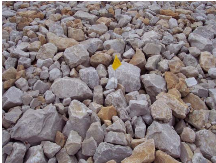
Photo 8. 2003-TP2; foot of north side slope of disposal cell.
