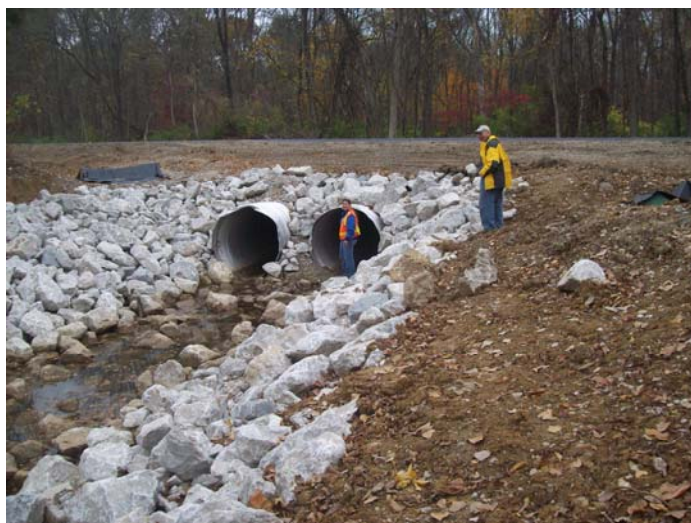
Photo 3. Hwy. D culverts outlet.
