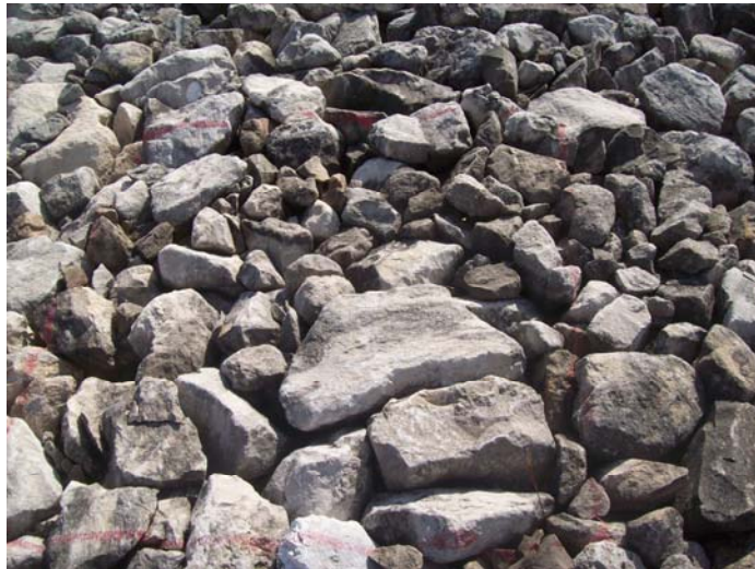
Photo 4. 2011-Cell cover test plot TP1; north edge of north facet.
