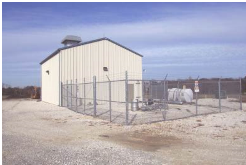
Photo 26: Outside of LCRS building.
