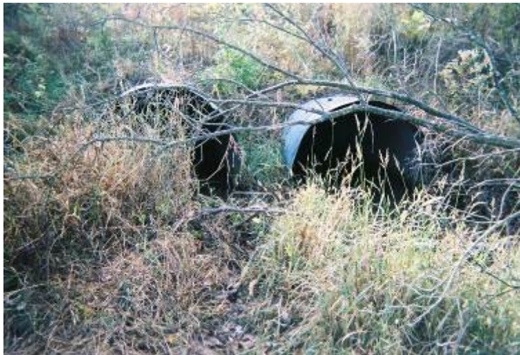
Photo 11: View of outlet side of twin culverts under Highway D.
