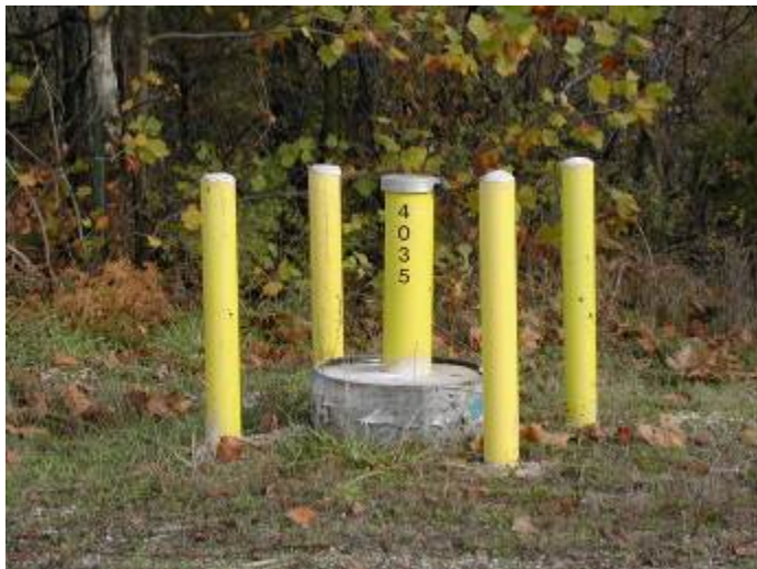
Photo 30: An example of a site groundwater monitoring well. This well is secured (locked), maintained, and properly identified.
