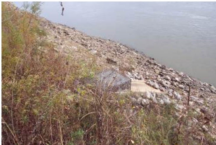
Photo 15: The weir that discharges from the LCRS Pipeline into the Missouri River.
