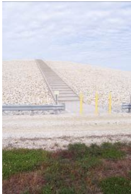
Photo 23: Stairs leading to the top of the disposal cell.
