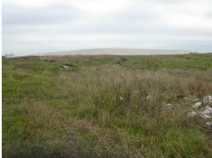
Photo 25: Erosion areas behind the disposal cell.
