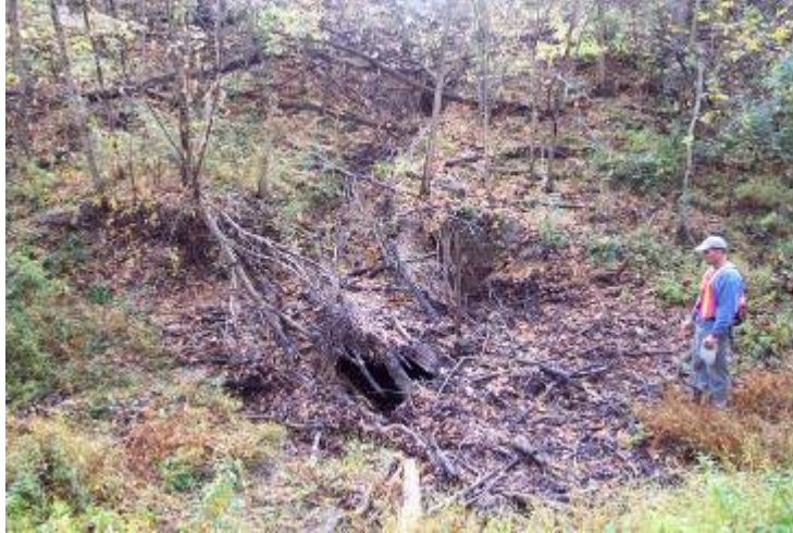
Photo 13: Inlet end of State Route 94 culvert.
