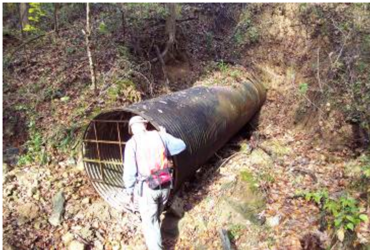
Photo 14: Outlet end of State Route 94 culvert.
