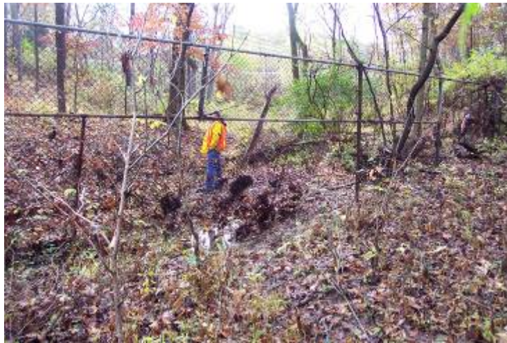
Photo 8: Fence across the Southeast Drainage upstream of Highway 94.
