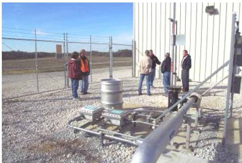
Photo 27: LCRS sump area with manhole in center of photo.
