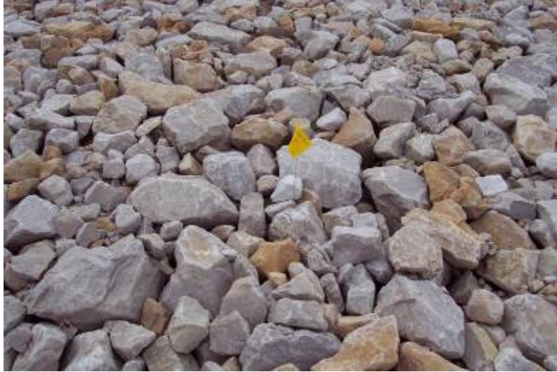
Photo 19: Test Plot 2 location for rock degradation information.
