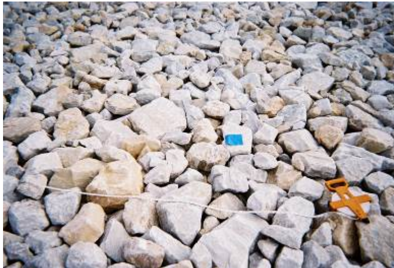
Photo 22: Test Plot 5 location for rock degradation information.
