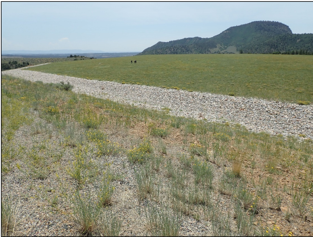
PL-6. Northeast Drainage Channel
