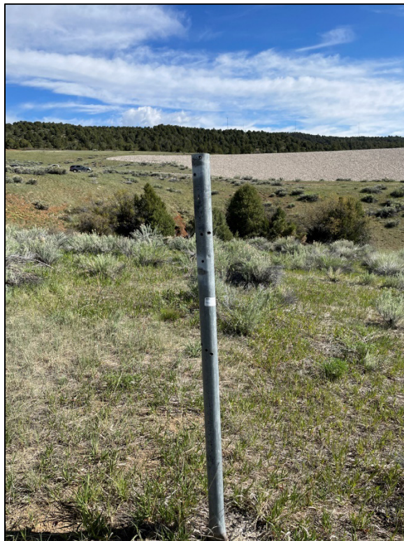
PL-2. Perimeter Sign P1 Missing
