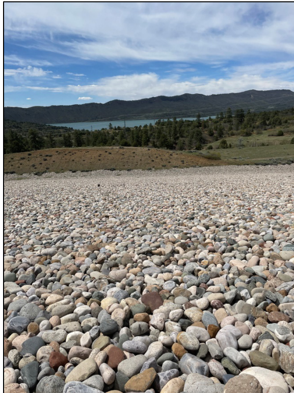
PL-9. South Side Slope
