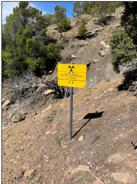
PL-4. Perimeter Sign P29 with Undercut Base but Stable
