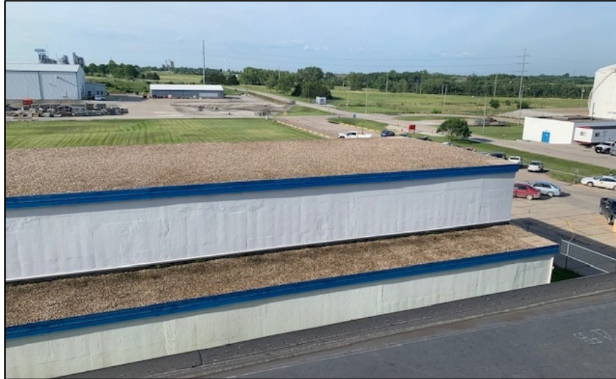
Photo 1. Roof of IHX Building
