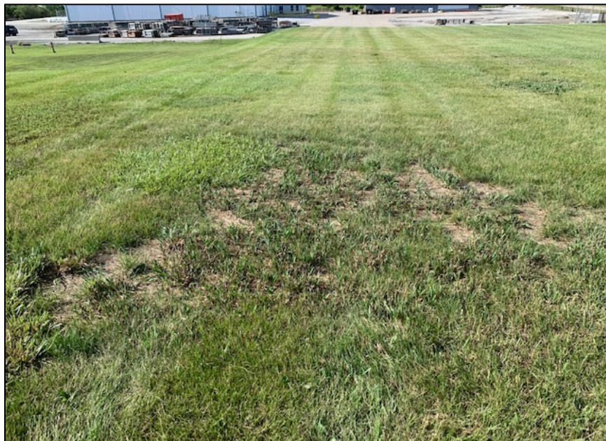
Photo 4. Condition of the Mound Grass (Poor)
