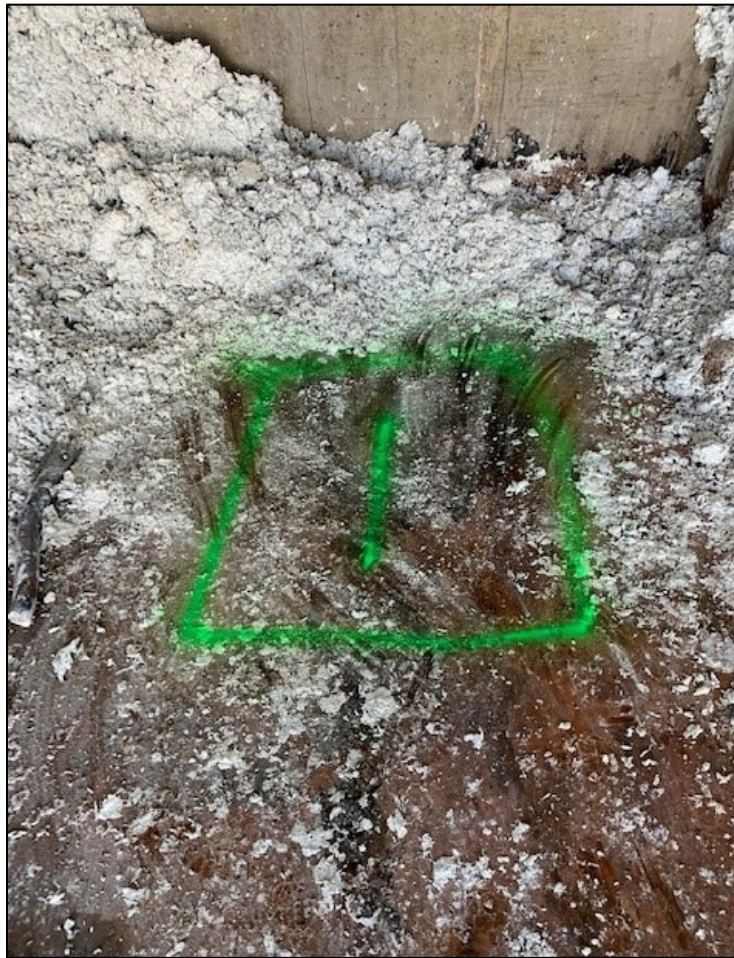
Figure 5. Survey Location No. 1, Room B-7 Floor
