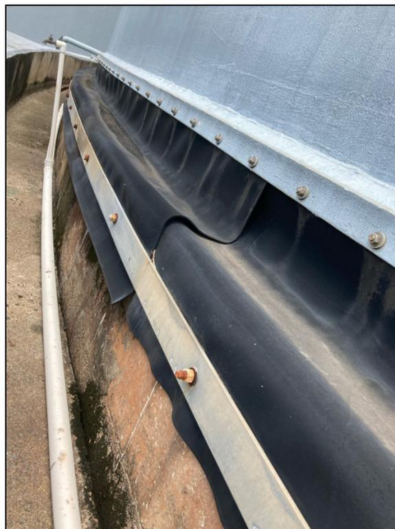
*PL-4. Gap in Seal at Base of Dome*
