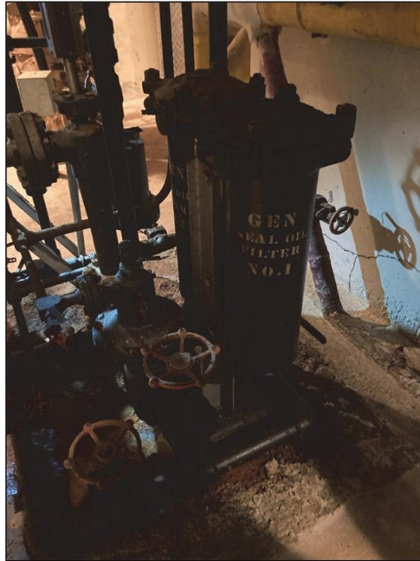
*PL-1. Oily Substance Noted at Base of Gen Seal Oil Filter No. 1*
