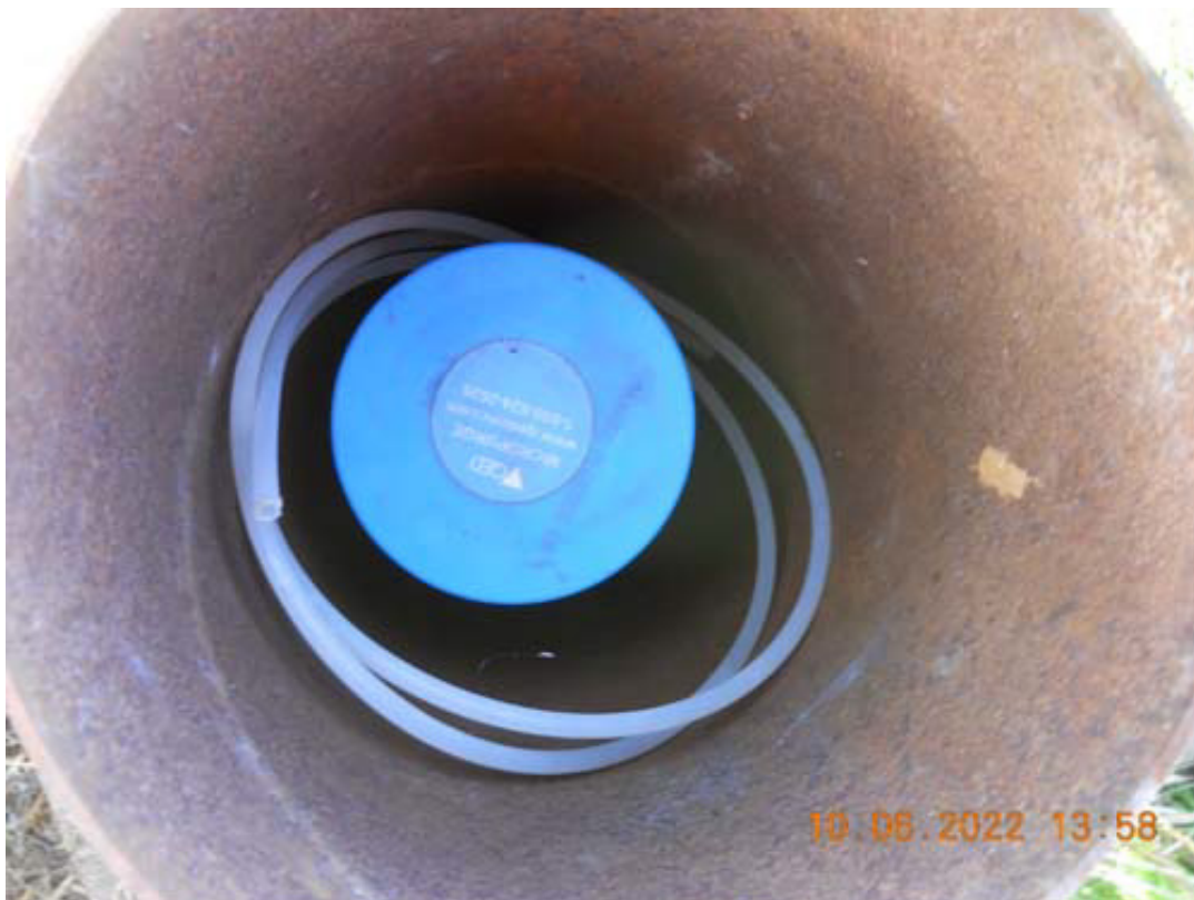
Well UCD1-018: Pump Manufacturer's Waterproof Cap Installed (Photo No. 4909)
