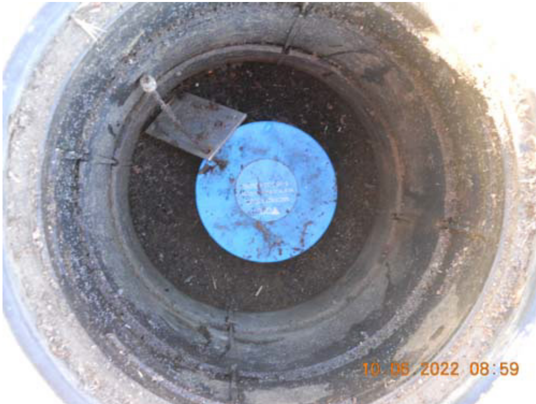
Well UCD1-023: Pump Manufacturer's Waterproof Cap Installed (Photo No. 4826)
