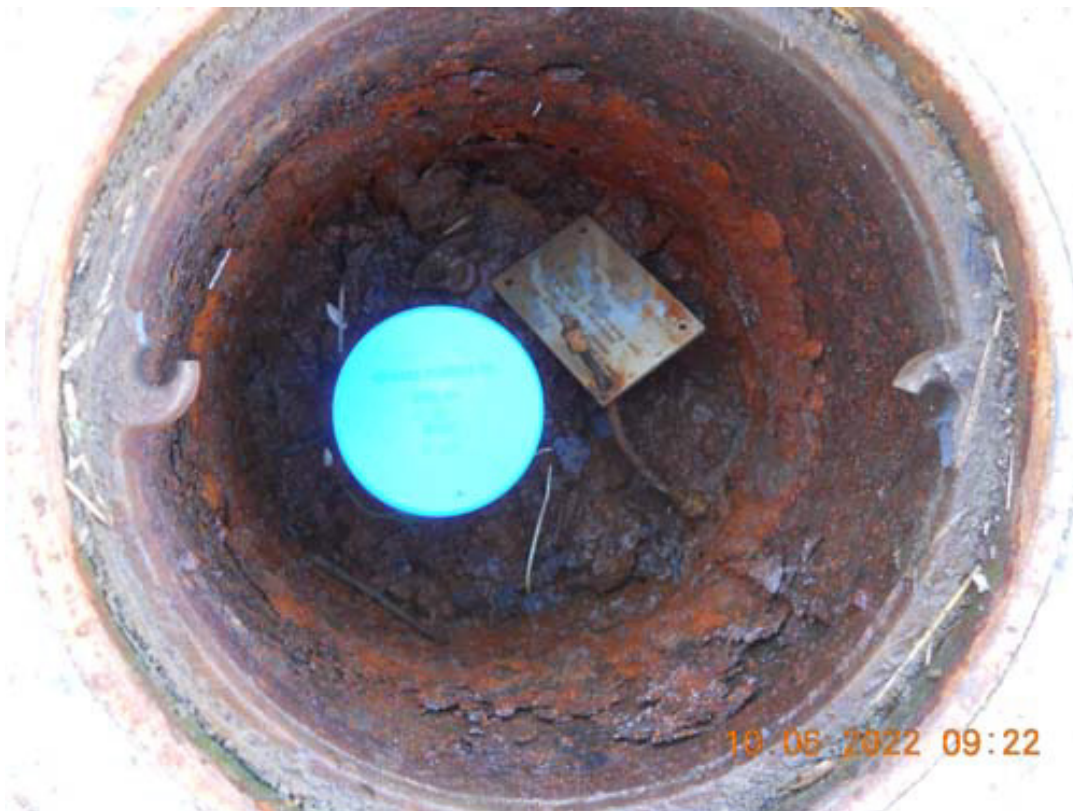
Well UCD1-072: Pump Manufacturer's Waterproof Cap Installed (Photo No. 4832)
