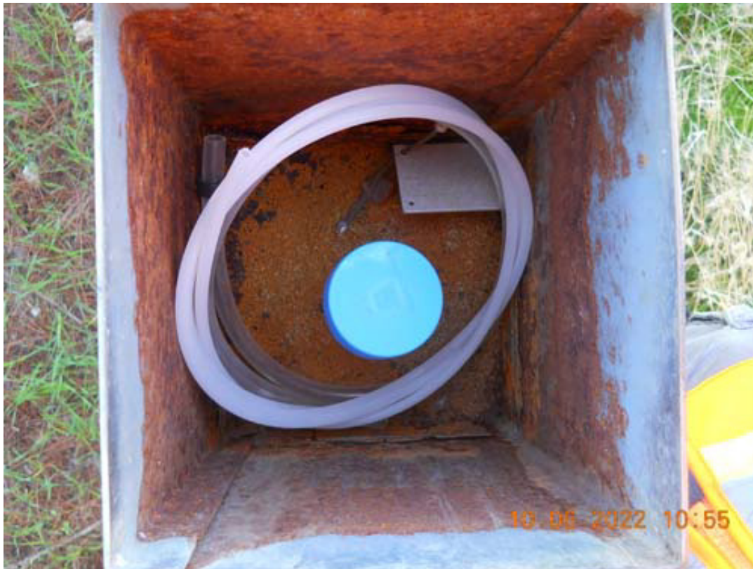
Well UCD1-070: Pump Manufacturer's Waterproof Cap Installed (Photo No. 4848)
