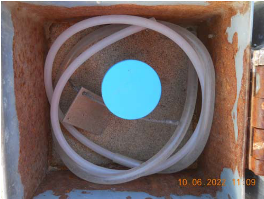
Well UCD1-063: Pump Manufacturer's Waterproof Cap Installed (Photo No. 4853)
