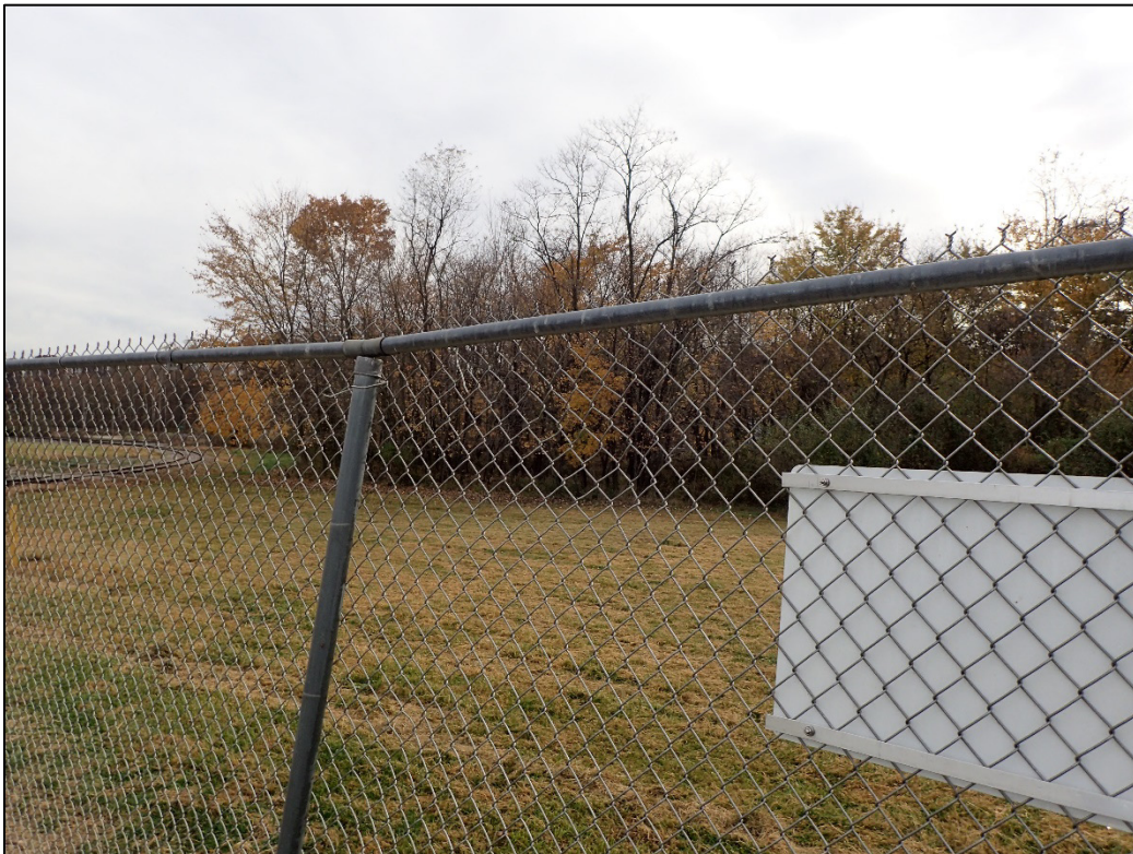
PL-4. Leaning Fence Post of Perimeter Fence
