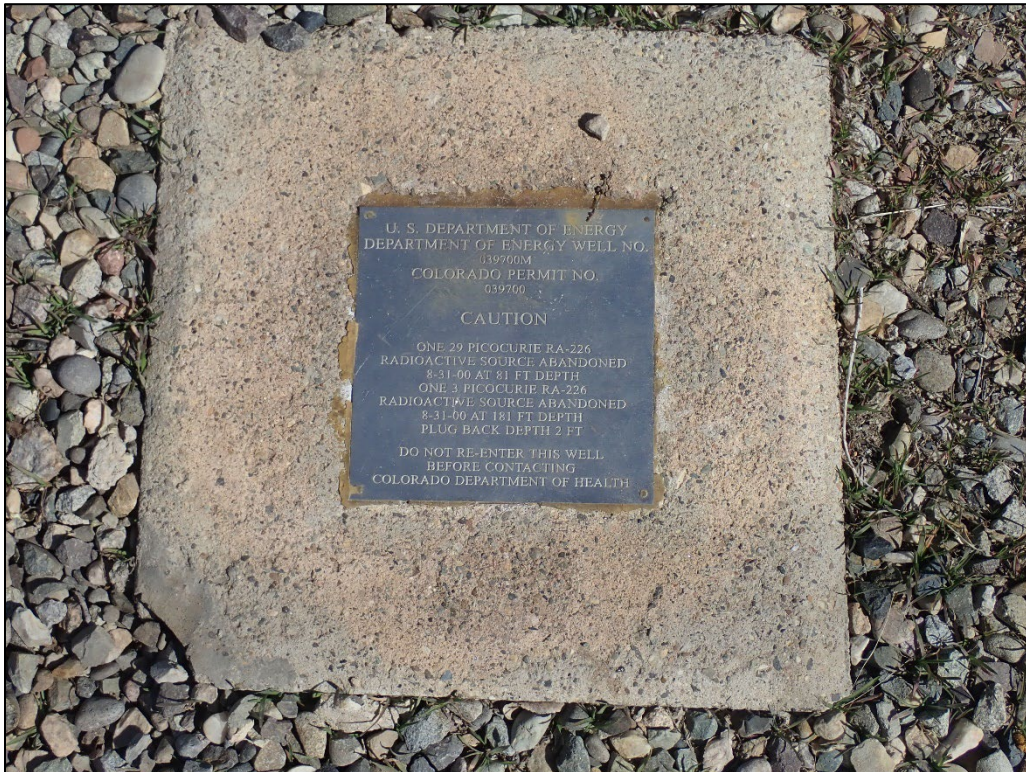
PL-6. Decommissioned Well Containing Radium Foil
