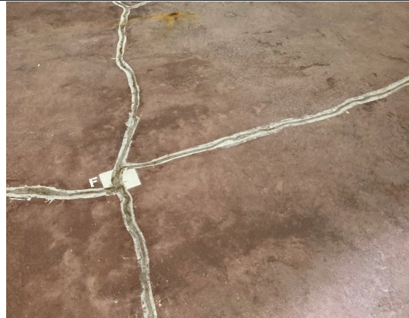
Figure 15. Closeup of Sealed Crack in the Red Concrete (1C-10)
