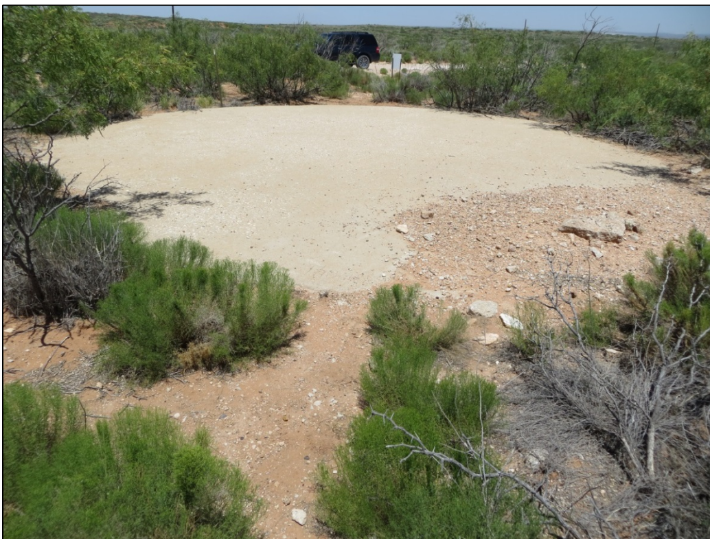
Looking northwest at the concrete cap that covers the Project Gnome emplacement shaft.
