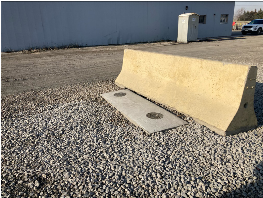
Photo 5. Flush-Mount Monitoring Wells OBS-7B and OBS-7C
