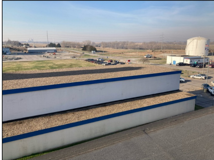
Photo 1. Roof of IHX Building
