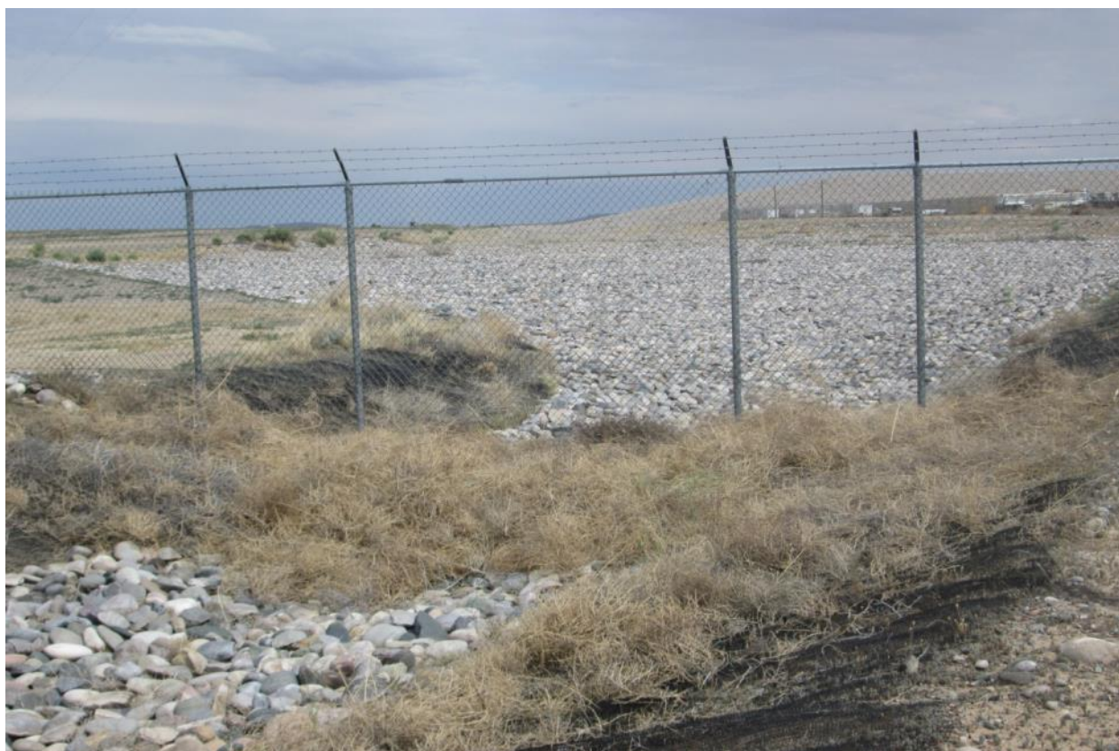
SHP 5/2014. PL-7. Tumbleweed accumulation in outflow channel.
