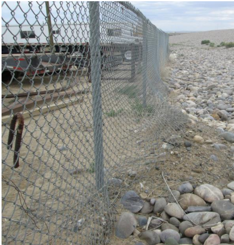
SHP 5/2014. PL-5. Dirt pushed through fence fabric between perimeter signs P11 and P12; no change from previous years.
