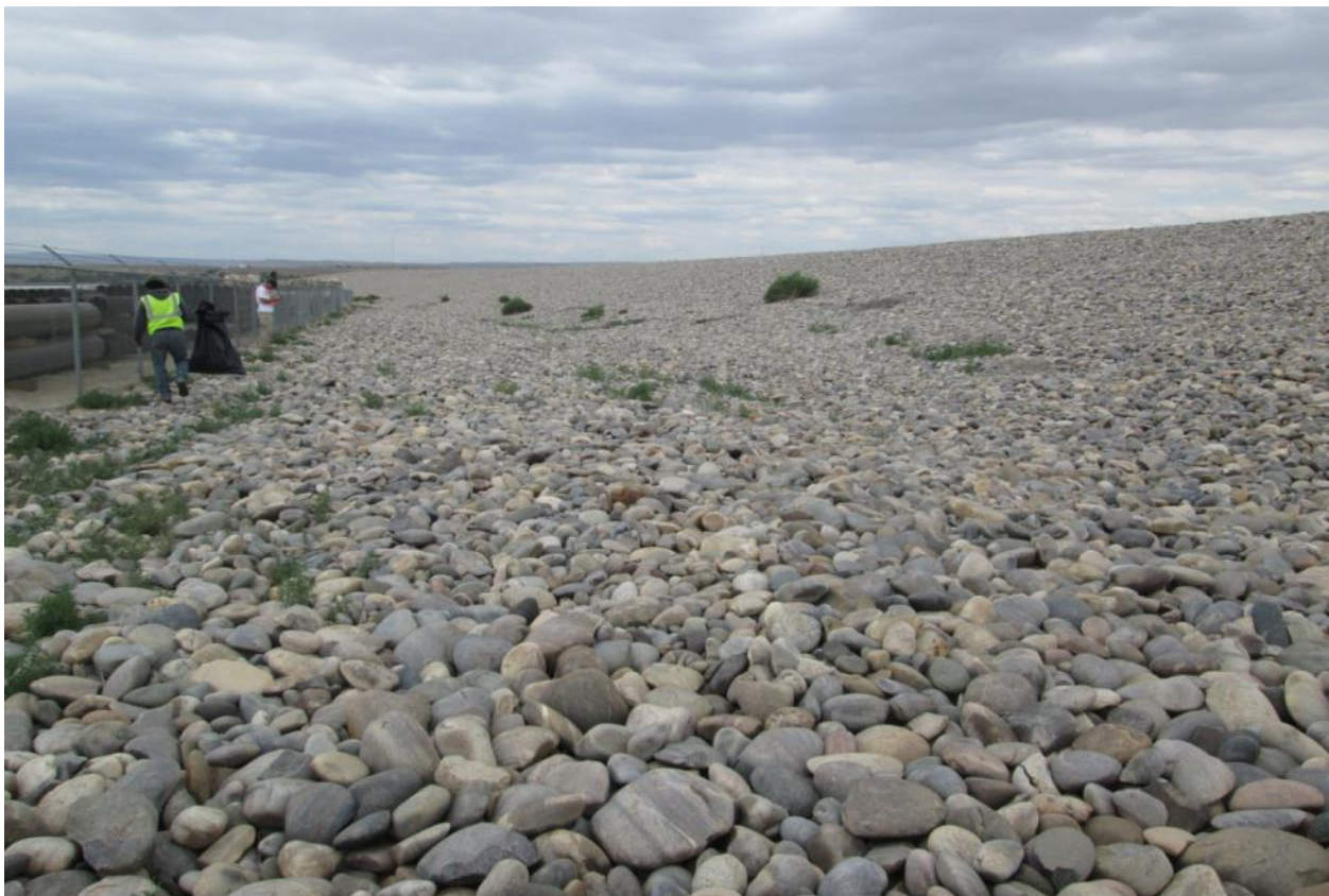
SHP 5/2014. PL-14. Diversion ditch and northwest side slope of disposal cell.
