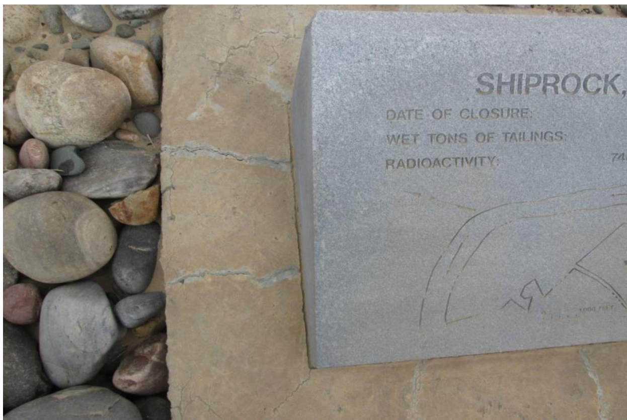
SHP 5/2014. PL-10. Repaired cracks in base of site marker SMK-1.
