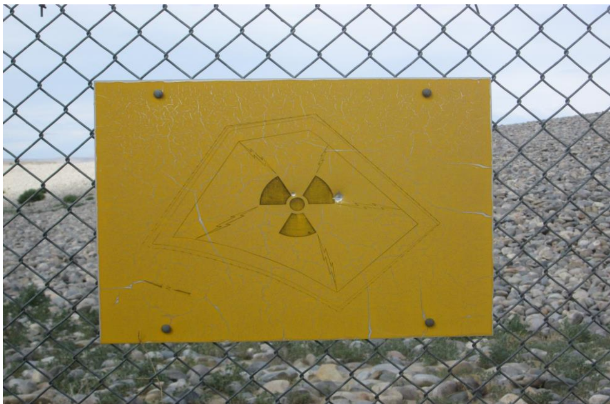
SHP 5/2014. PL-4. Bullet holes in west entrance pictorial sign; note cracked and faded surface.
