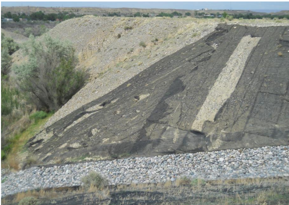
SHP 5/2014. PL-16. Loose erosion control fabric along outflow channel side slope.
