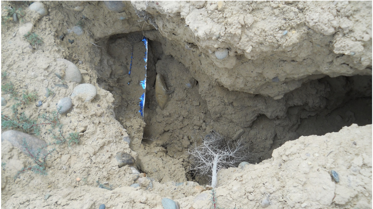
SHP 5/2015. PL-13. Soil erosion exposing buried water pipeline.
