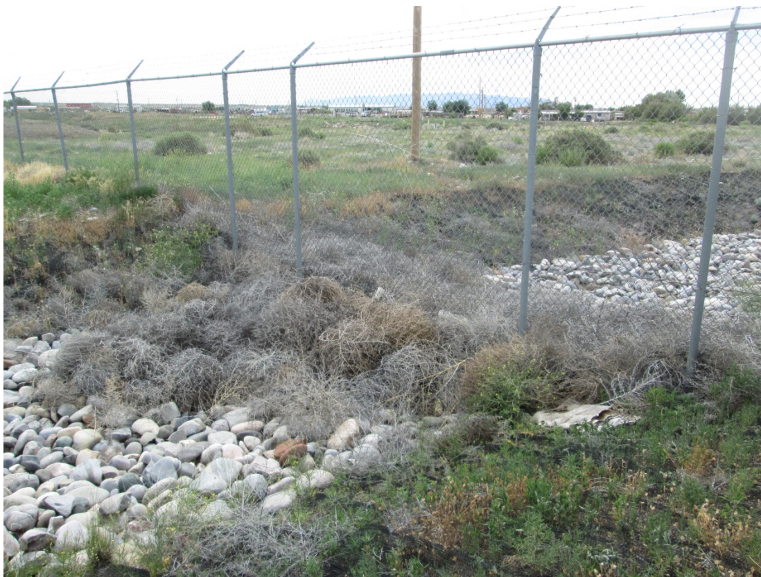
SHP 5/2015. PL-7. Tumbleweed buildup in outflow channel next to perimeter fence.
