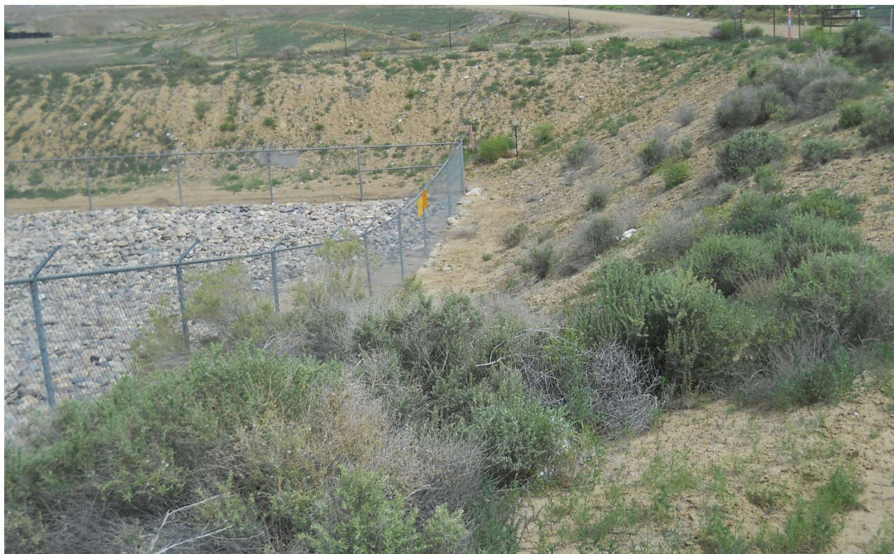
SHP 5/2015. PL-11. View of eroding slopes adjacent to the southeast and southwest perimeter fences.
