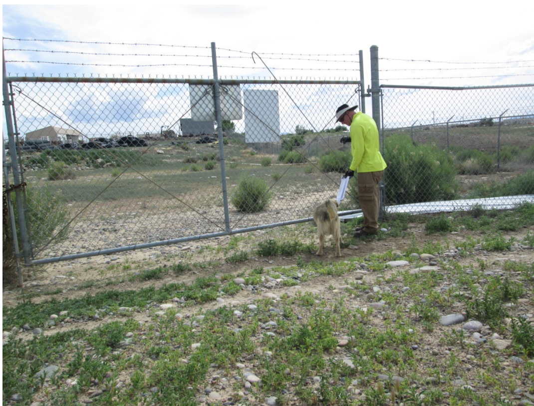
SHP 5/2015. PL-1. View of 12-inch gap under north gate before repair; the gap allowed trespass by local dogs.
