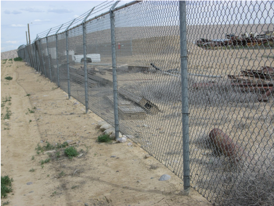
SHP 5/2015. PL-5. Perimeter fence with 3- to 6-inch gap on bottom.
