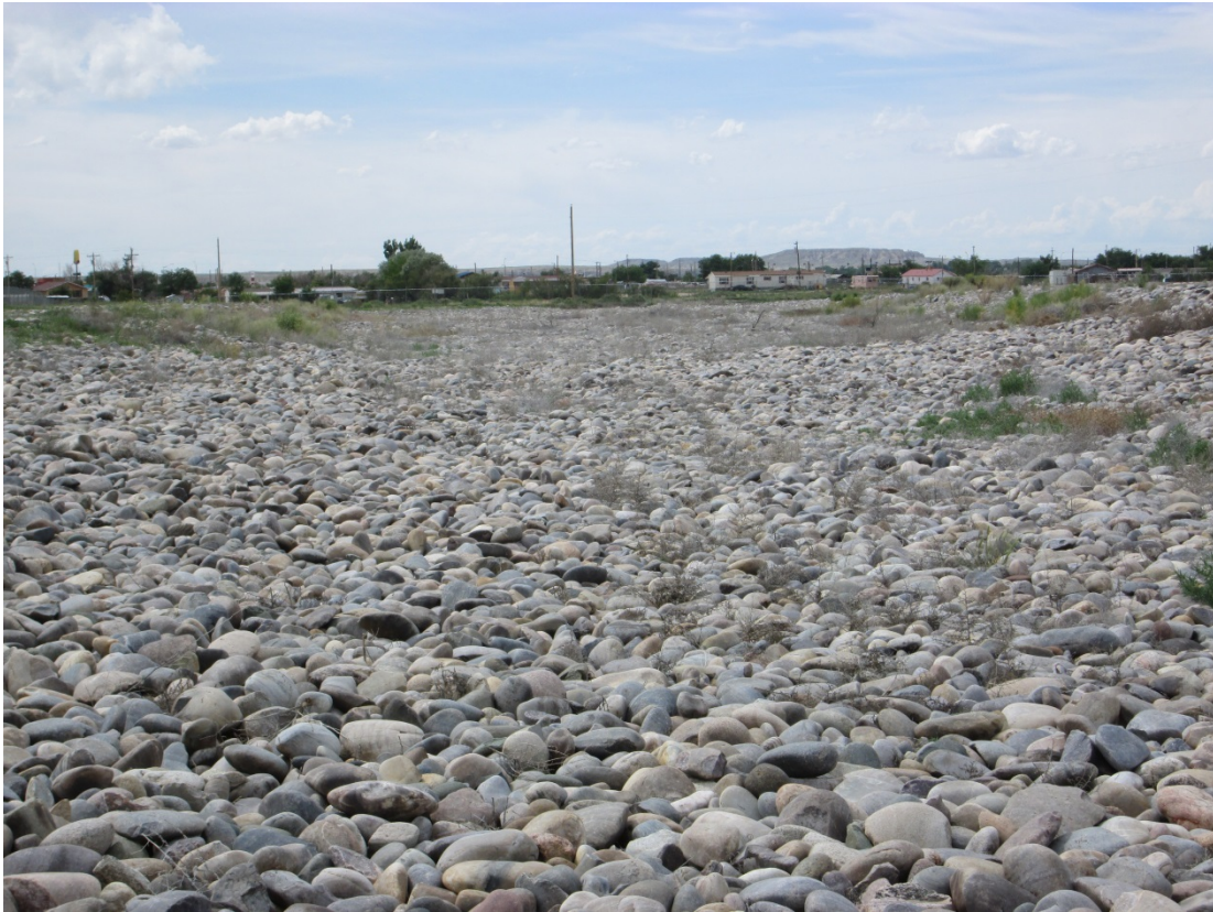
SHP 5/2015. PL-9. Unobstructed outflow channel.
