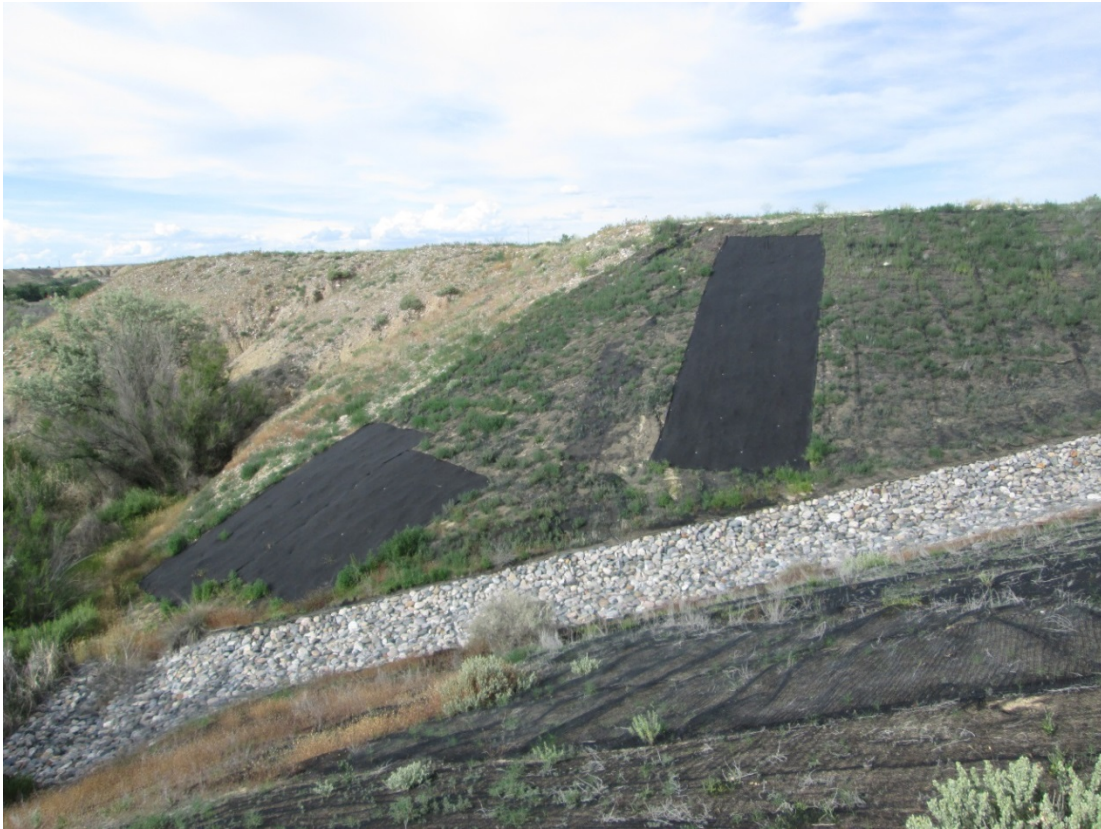
SHP 5/2015. PL-15. Recent repairs to erosion control fabric on lower end of outflow channel.
