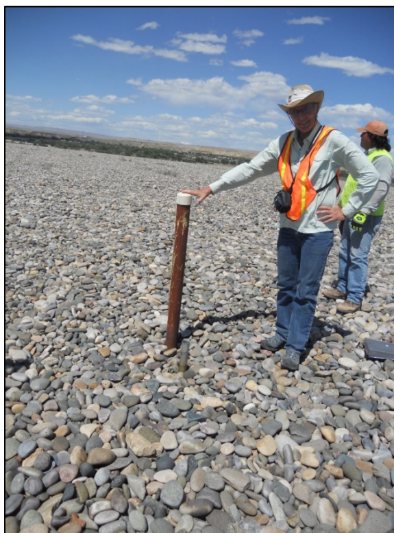
PL-8. Historical Neutron Hydroprobe Port on Disposal Cell Top Slope
