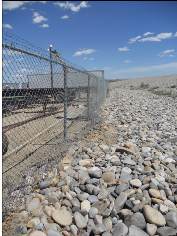
PL-1. West Perimeter Fence Along NECA Yard; Note Historical Damage to Fence Fabric
