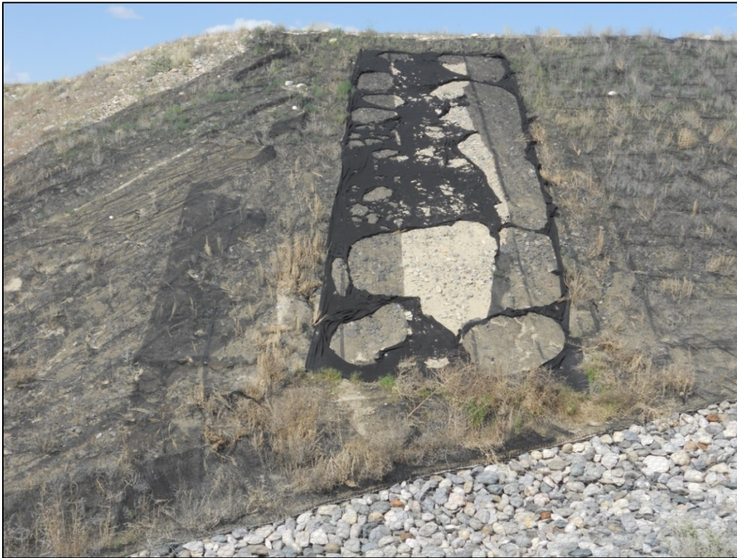
PL-13. Damaged Erosion Control Fabric on Upper Part of Outflow Channel Side Slope
