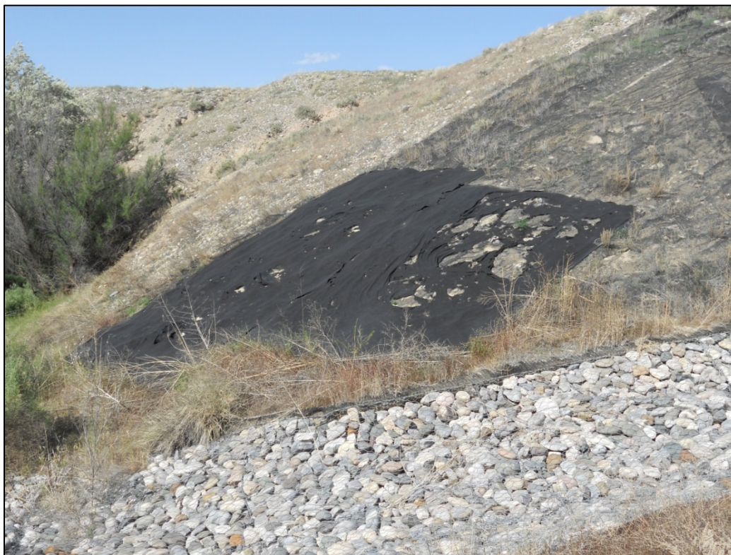
PL-12. Damaged Erosion Control Fabric on Lower Part of Outflow Channel Side Slope
