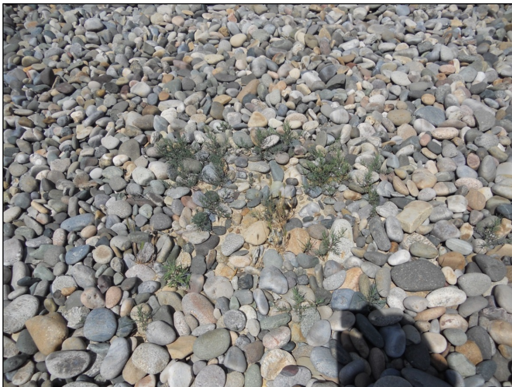
PL-7. Typical Annual Weed Cover on Disposal Cell Top Slope
