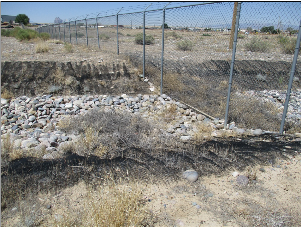
PL-4. Tumbleweeds in Outflow Channel at Perimeter Fence
