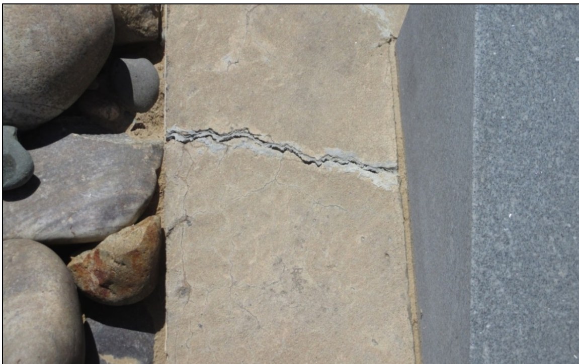
PL-7. Crack on Site Marker SMK-1 Concrete Base (Repaired Following Inspection)
