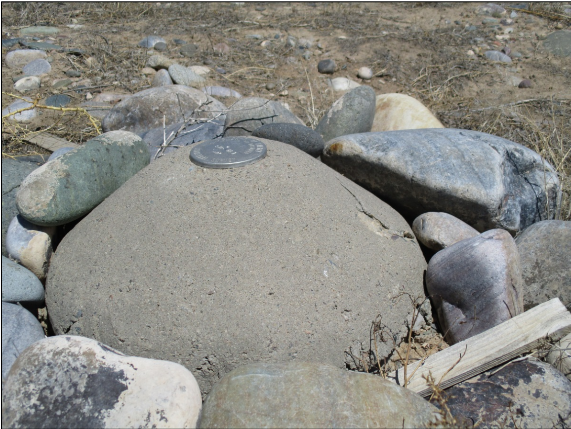
PL-9. Crack in Base of Survey Monument SM-1
