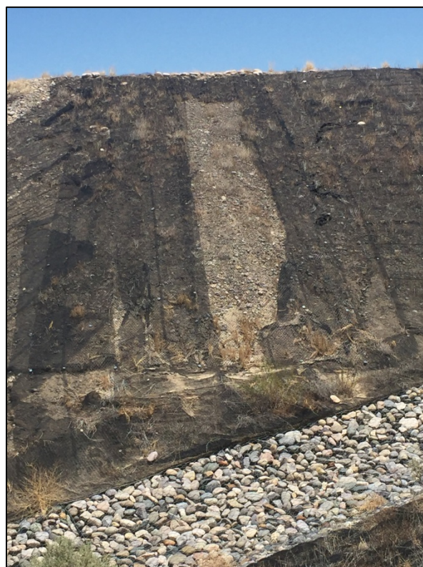
PL-12. Damaged Erosion Control Fabric (Need for Repair to Be Evaluated)
