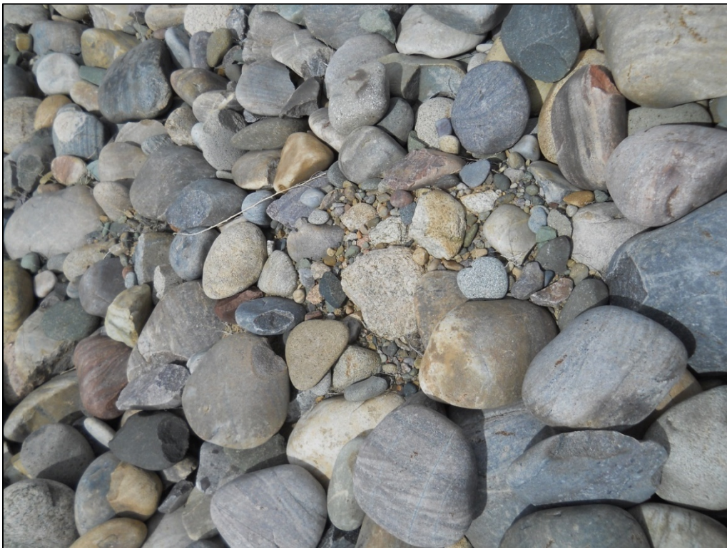
PL-6. Exposure of Smaller Cobbles and Gravels Along Ridge of Disposal Cell
