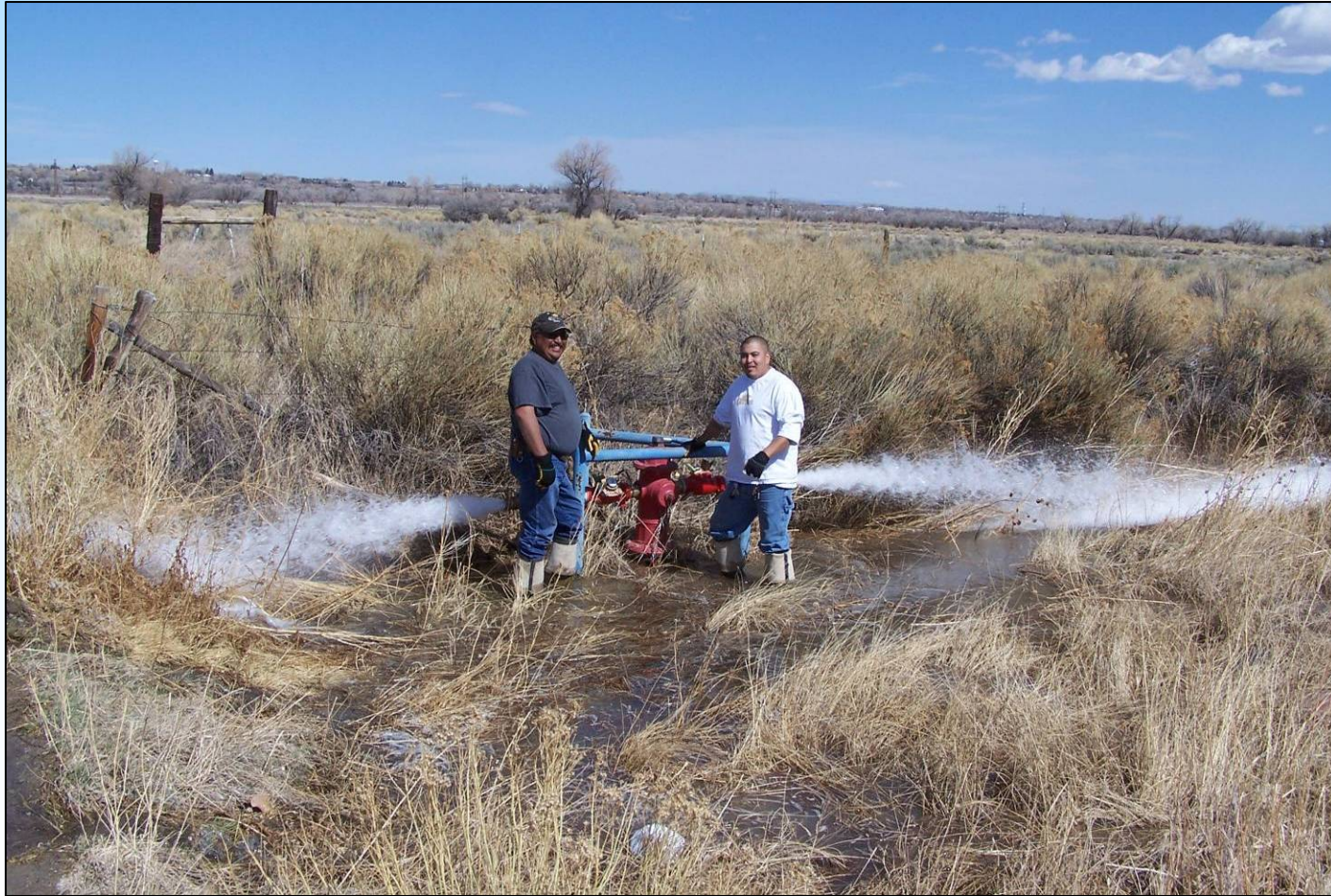
Northern Arapaho Utility Organization Hydrant Flushing
